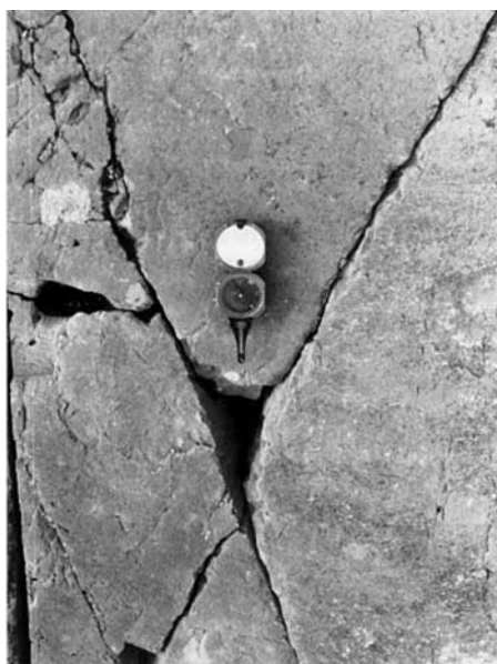
Fig. 10. Conjugate set of shear fractures in limestone block of temple floor (see Fig. 8).
