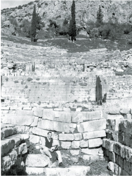
Fig. 12. Collapsed segment of SW part of the Apollo temple, which is also the area with the greatest density of shear fractures (Fig. 11). Collapse probably resulted from same stress field as that represented by the fractures and indicates the former presence of a space (adyton?) below the temple floor.
