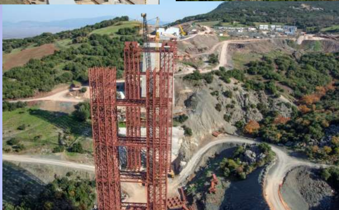
RAILWAY BRIDGE 26 (409 m LONG)
