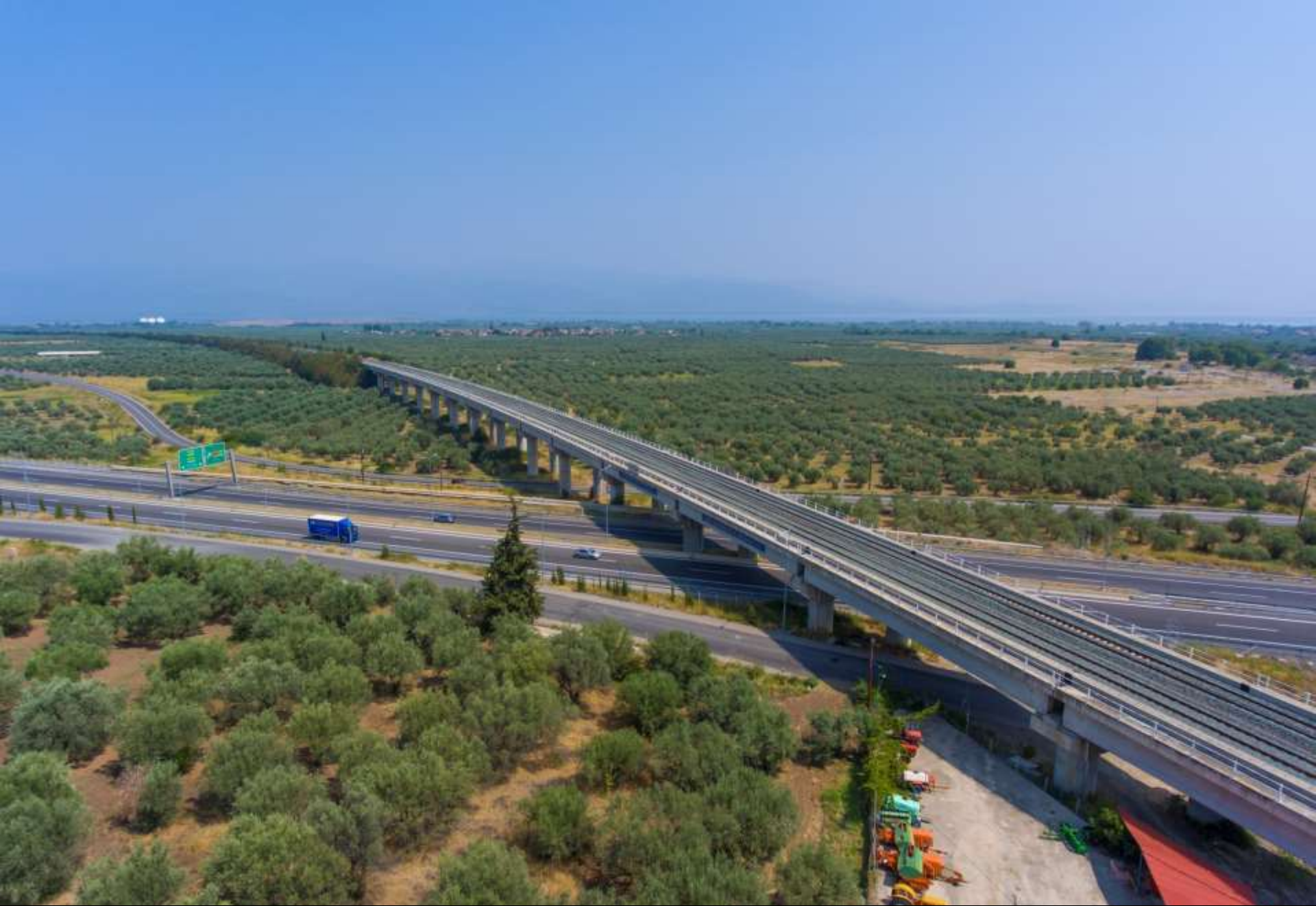
RAILWAY BRIDGE OVER NATIONAL HIGHWAY (500m LONG)
