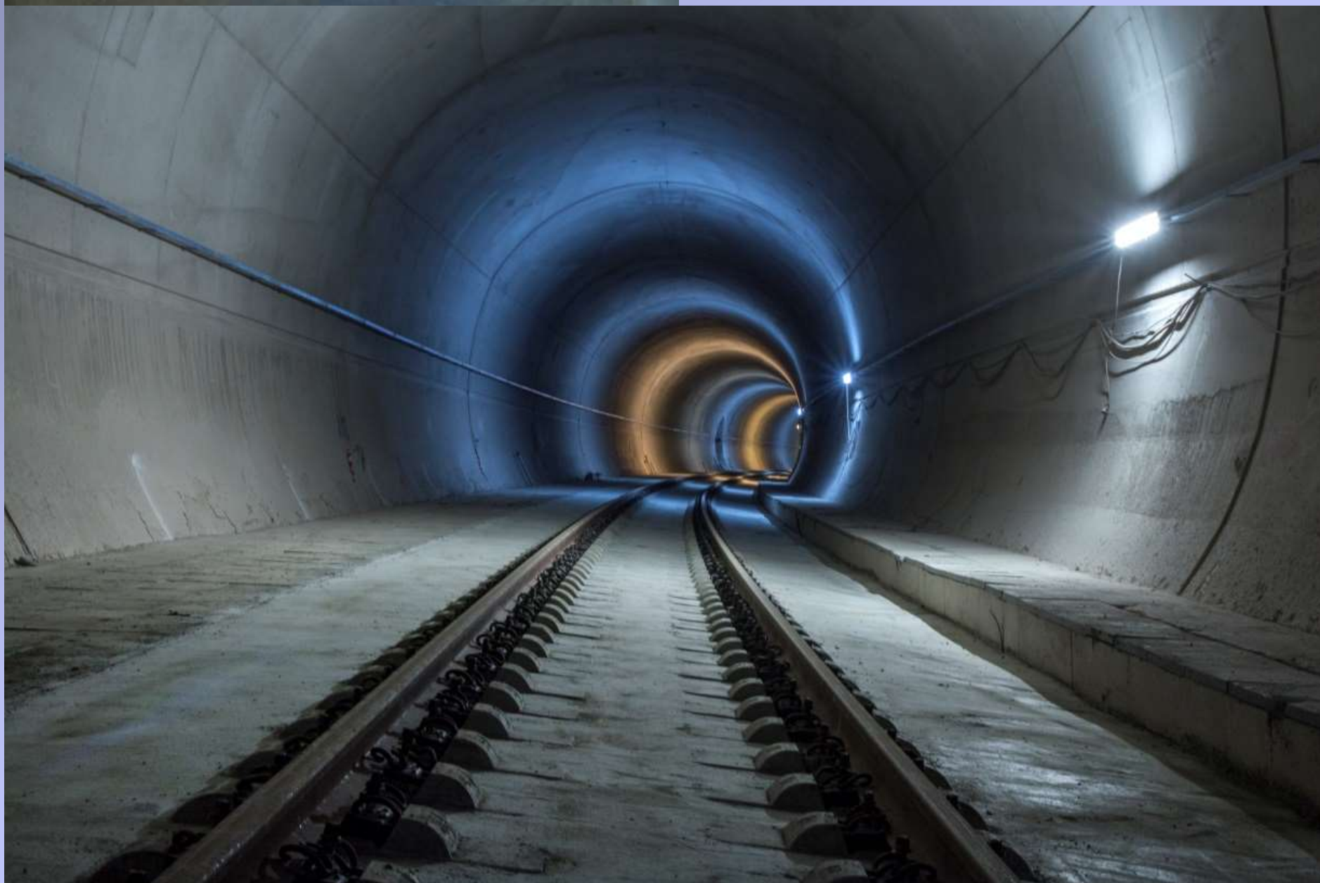
OTHRYS TUNNEL – each tube 6,4 km long
