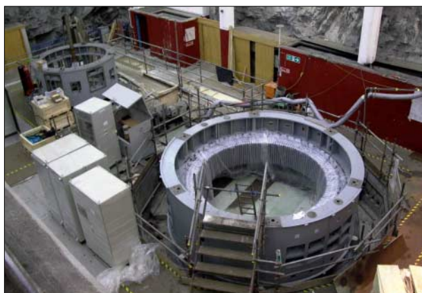
Shot of the refurbishment at Ceannacroc (20 MW), by Fort Augustus. It was accredited for ROCs in April 2003.
