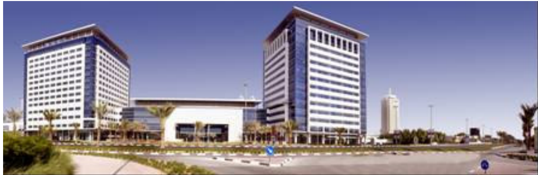
Figure 4.1 DWTC Office Block Image
