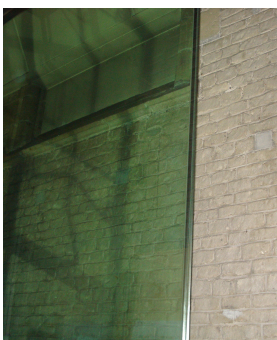
Fig. 8. The green glass enclosure
