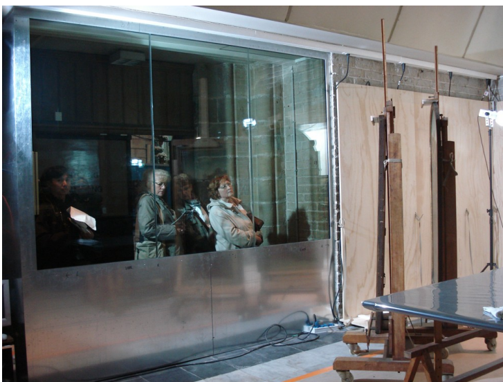
Fig. 3b. Glass wall separating the Villa Chapel from the visitor gallery
