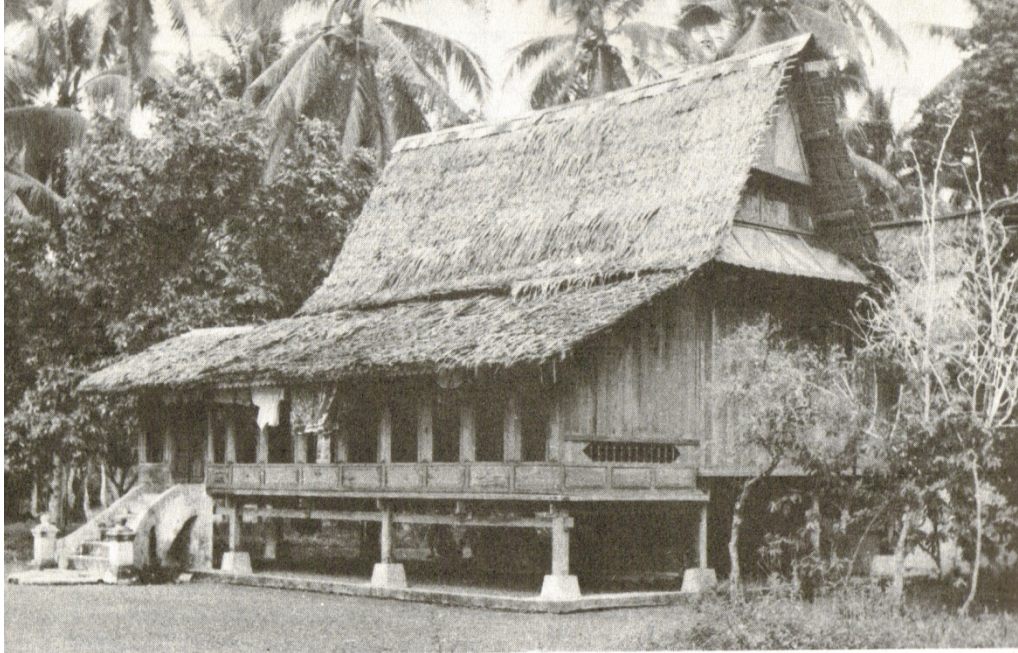
Fig. 2.33—MALAY HOUSE, MALACCA (2°14'N.). Traditional Asian design for a hot humid climate (day temperature 88°-98°F., night 72°-73°F., vapour pressure 32-33 m. bars). Note the low-eaved verandah giving protection against sky glare as well as rain.
