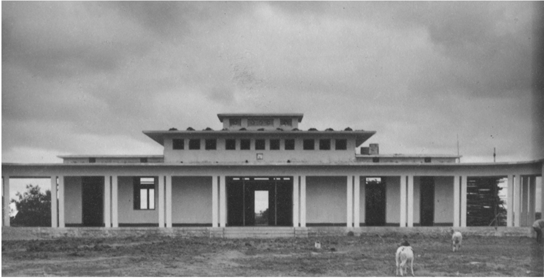
Figure 2.22 The Front Elevation of the Serum Institute, Hebbal, Bangalore, 1942. Source: Otto Koenigsberger's Portfolio, OKPP.
