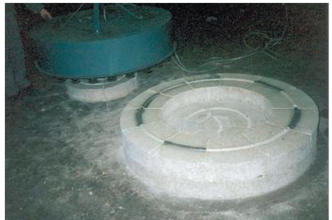
Fig. 13.- Arrangement of compacted bentonite blocks to be placed in an experimental vertical shaft (Astudillo et al. , 1993).
