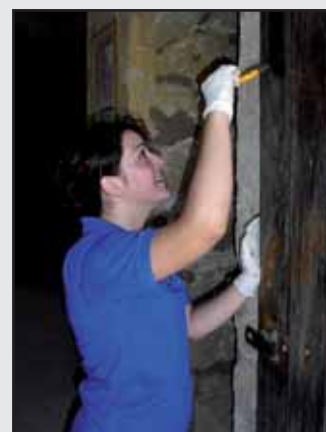
Jantess applying lacquer to the door of Dwejra Tower
