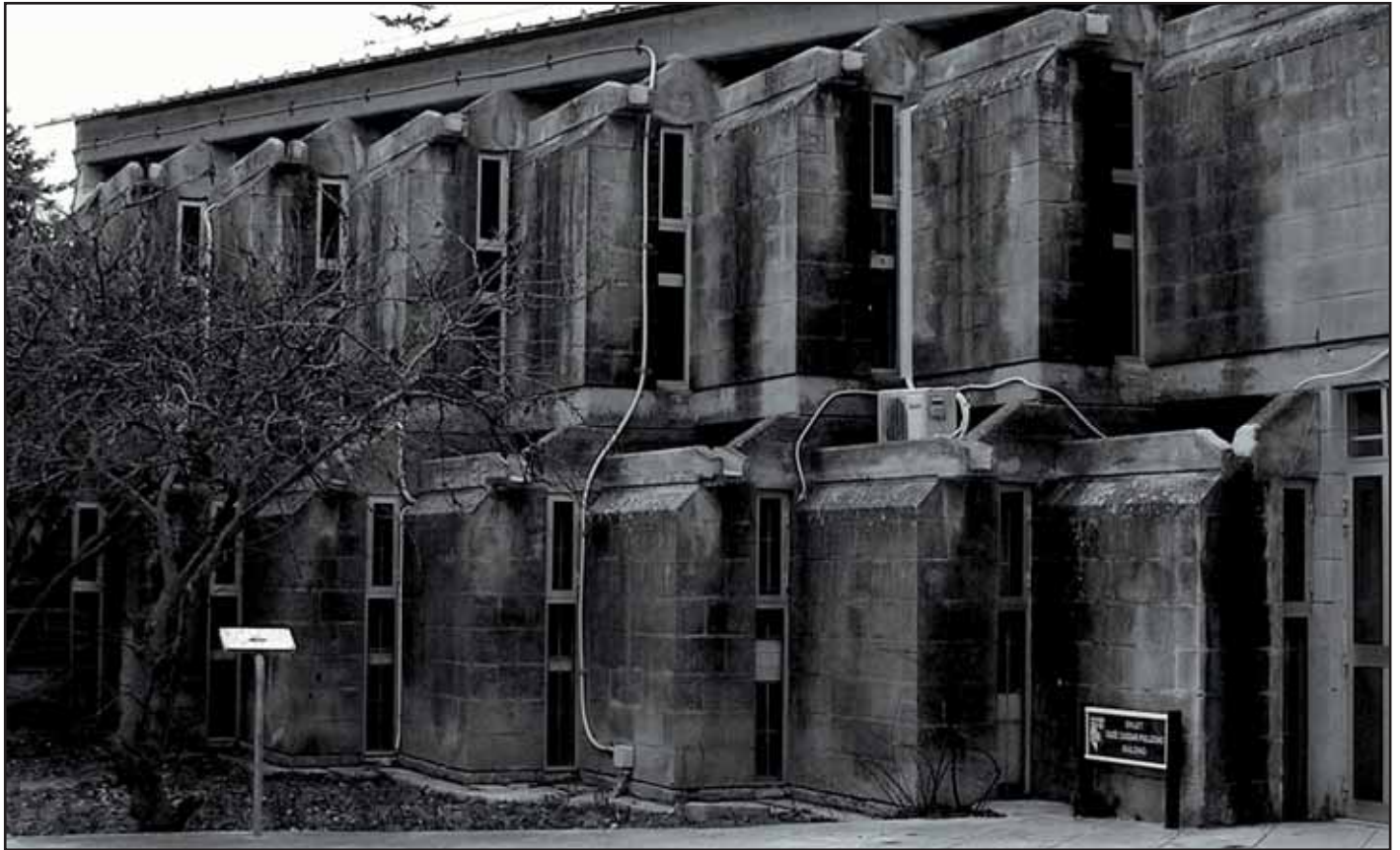
Former Faculty of Architecture building, University of Malta
