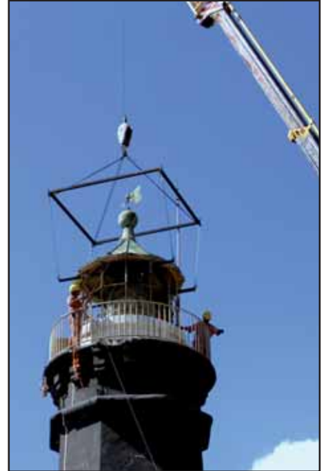
Preparing to lower the housing
