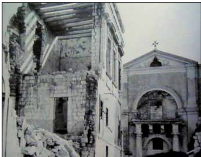
Bomb-damaged site in front of St John’s Co-Cathedral by Alfred Vella Gera
