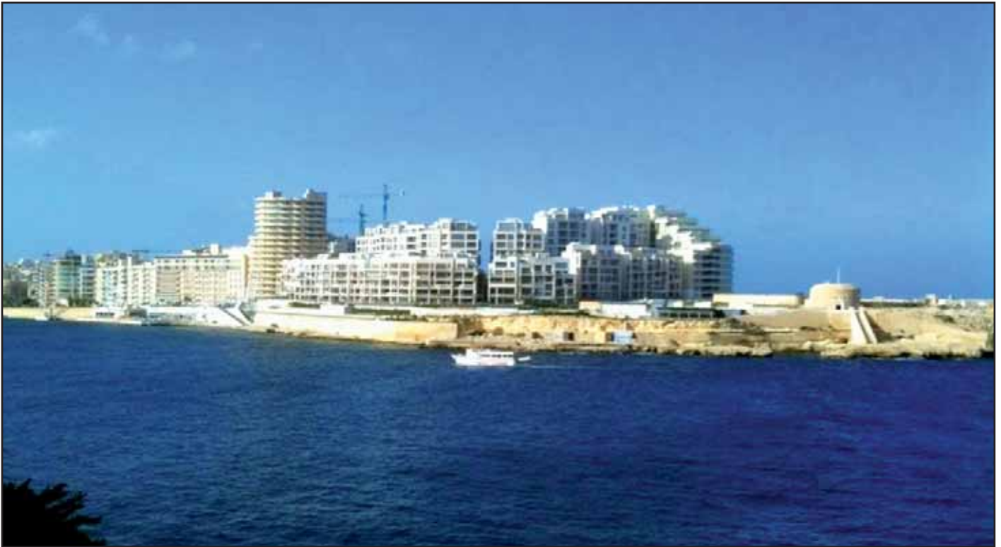
Built only for people looking out
