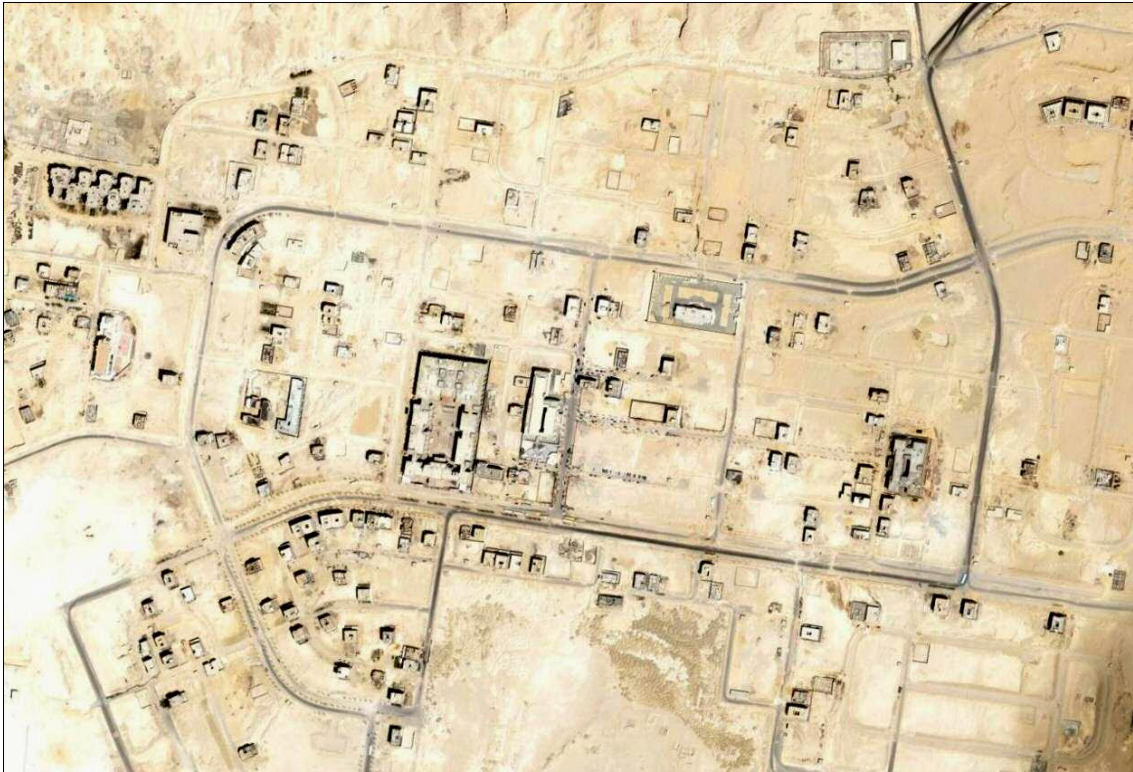
Figure 6: Example of stalled subdivision development (Muqattam Middle Plateau, started in 1979), Google/DigitalGlobe Image (from 2005)
