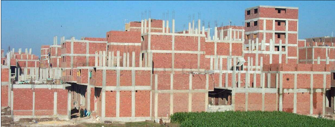
Figure 15: New Informal Housing, Giza
