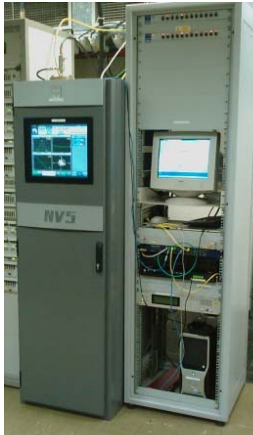
Figure 7: The DRM+ transmitter (left) and content server, modulator and monitoring receiver (right)
