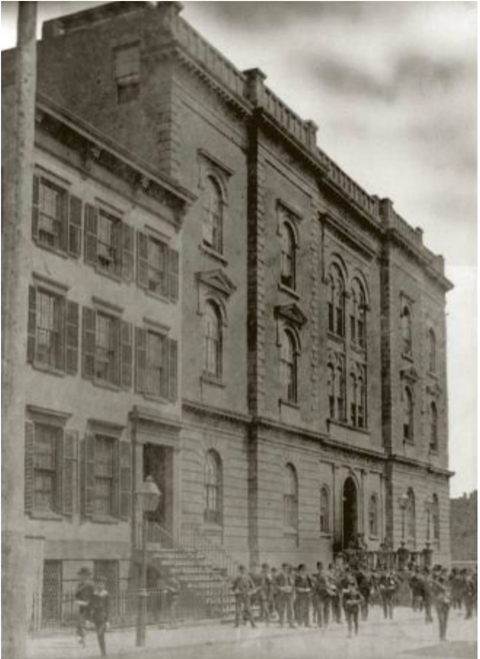
The 99 Livingston Street building in the late 1880s. Some Preparatory School students can be seen in knickerbockers on the far left, while older Collegiate Department students are on the right.
