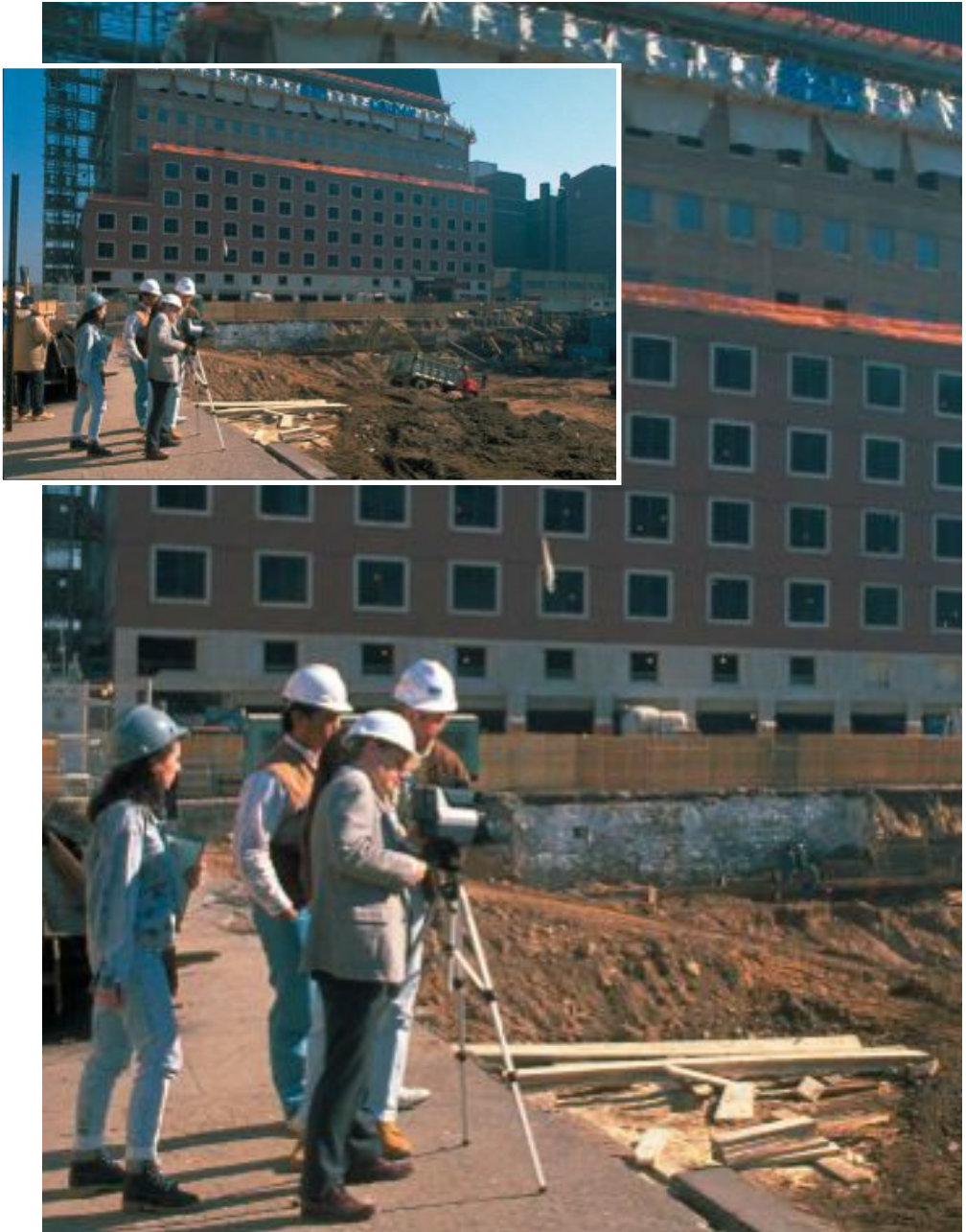
The development of MetroTech represents the vision, brought to life in concrete, steel, and stone, of George Bugliarello for a better Polytechnic University and a renewed downtown Brooklyn. This picture shows early work on the MetroTech construction site.
