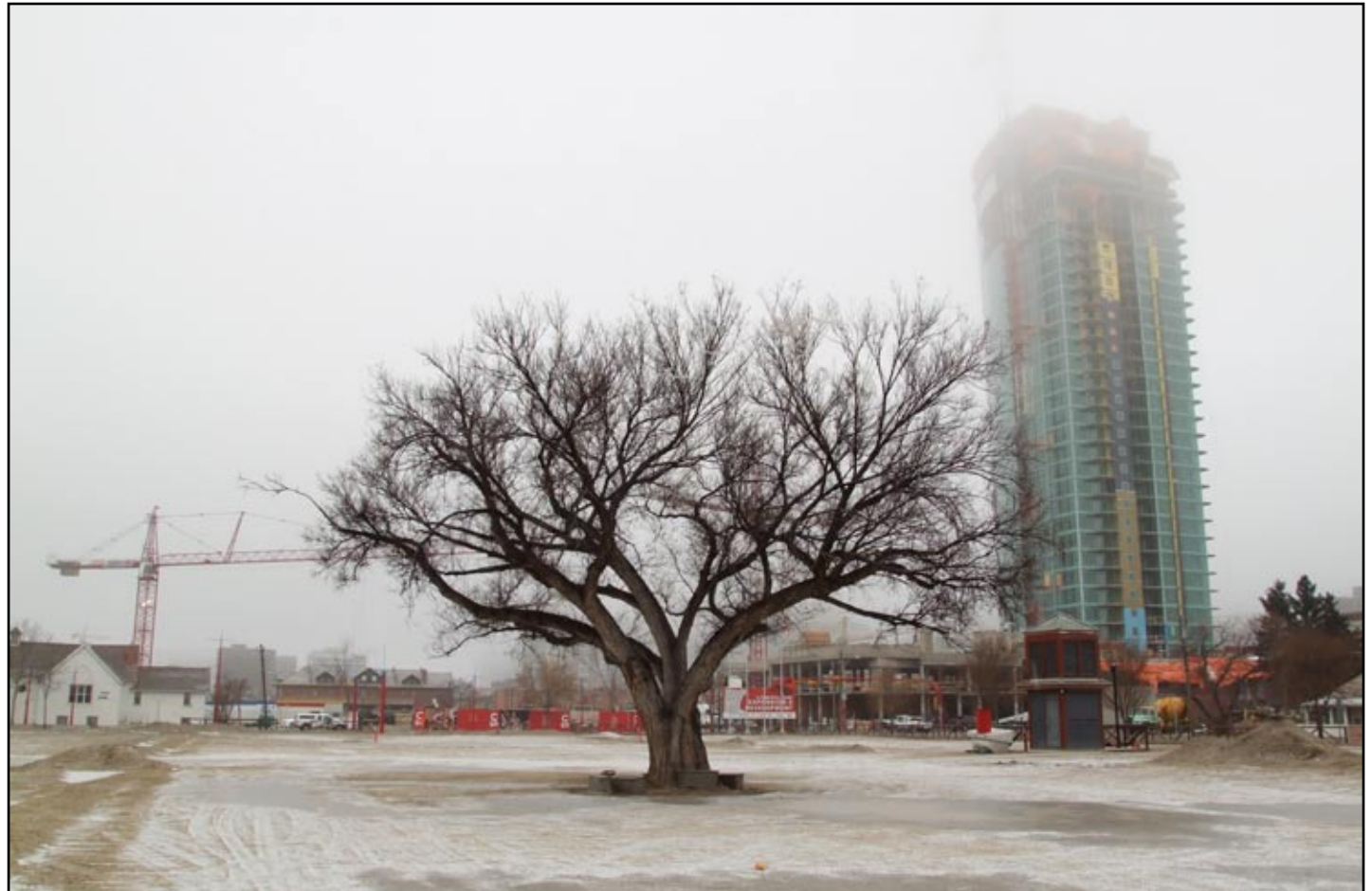
Site of former low income rental housing razed for development in Victoria Park. "The eye-popping price growth in Calgary (reaching gains of 50 per cent to 60 per cent) is simply unsustainable," reports the CMHC.
