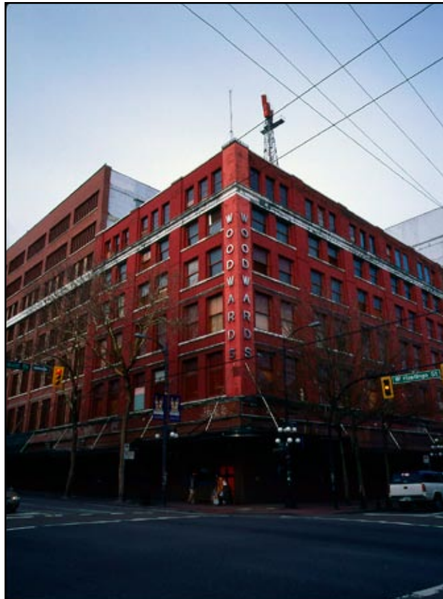
Renewal in Vancouver’s Downtown Eastside: the Woodward’s project with 200 units of affordable housing to be built amid 536 market-priced units
