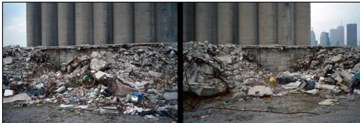
Toronto: site of former Rooster Squat, a homeless camp inside abandoned concrete silos.
