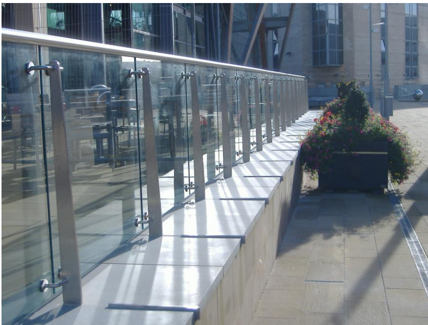
Figure 8: Wall detail, Millennium Square, Sheffield
