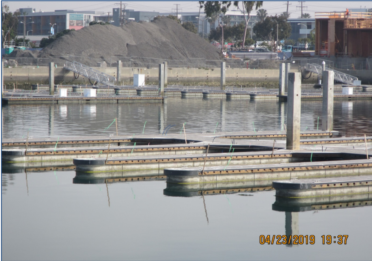
Photograph 16. Wooden poles and lines used to suspend flagging in Basin G in Marina del Rey Harbor.
