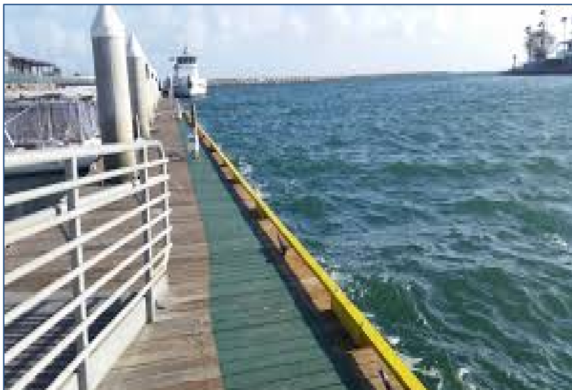
Photograph 12. Wood bull rail on dock in Port of Long Beach.
