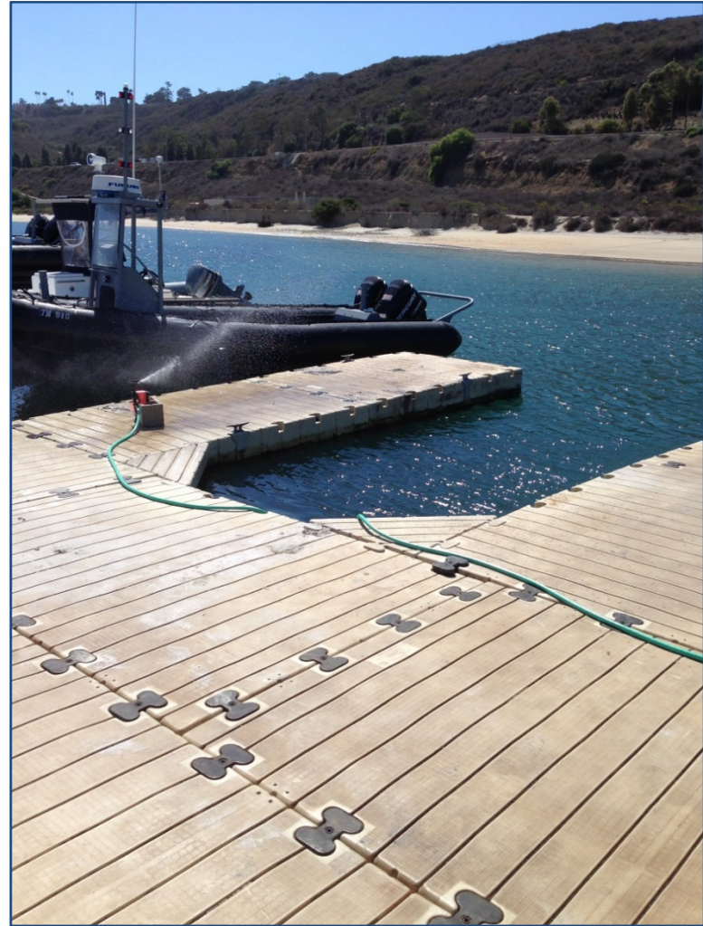
Photograph 21. Sprinkler with motion detector in operation at Navy Base Point Loma, Point Loma, California.
