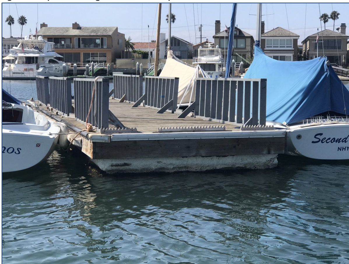
Photograph 13. Wood exclusion barrier and wood spike strips on a dock in Newport Beach (Source: The Log).
