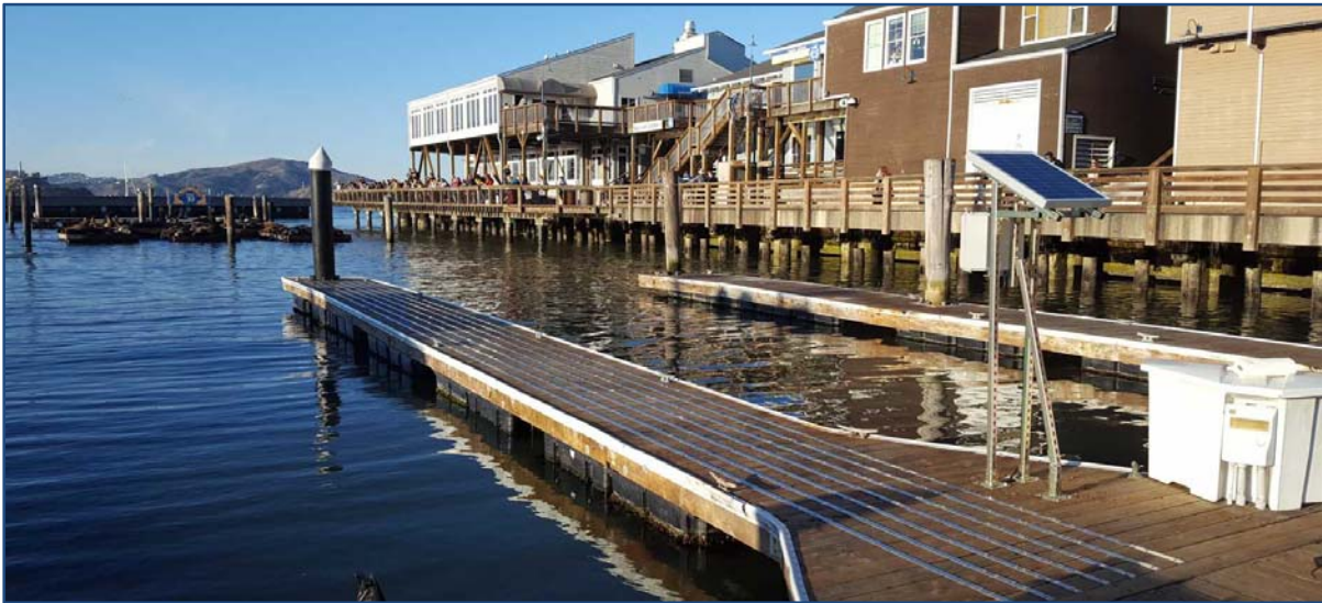
Photograph 14. Smith-Root’s Pinniped Deterrence System in Pier 39, San Francisco, California (Source: Smith-Root’s website 2019)
