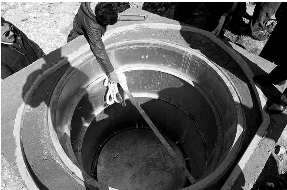
Fig. 7.40 Interior of a seismic vault made of welded metal sheets. The vault is big enough to accept weak- and strong-motion instrumentation together with data acquisition and transmission equipment.
