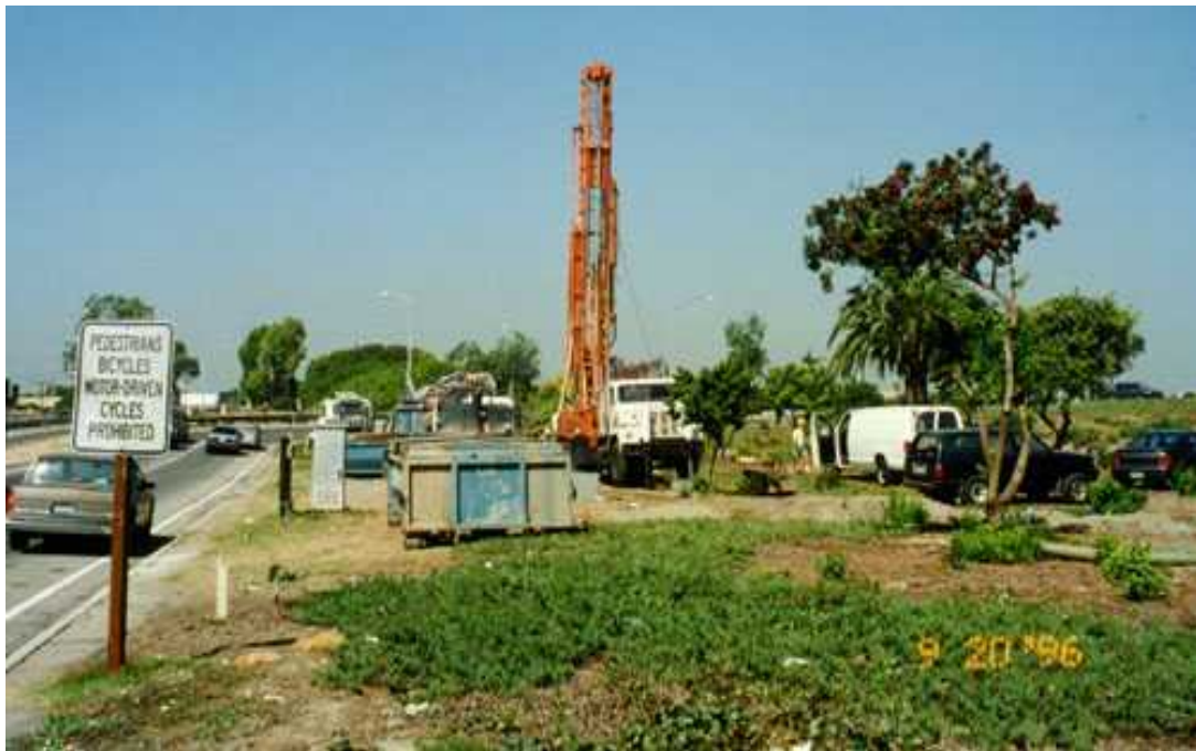
Fig. 7.66 Typical borehole drilling operation in an open area.
