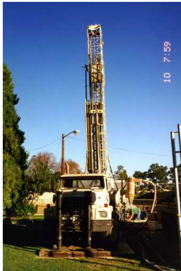
Fig. 7.67 Drilling operation in a confined area, showing size of drill rig.
