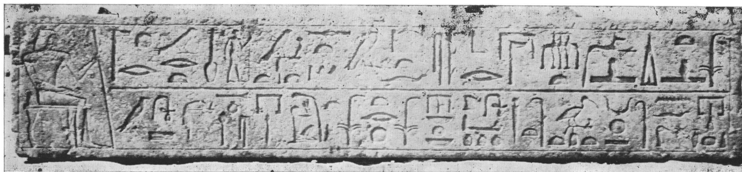
The lintel of the entrance
