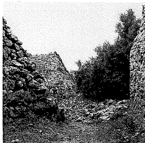
Going back down we spent time in the village, and here again was magic. The houses, made of field stone, piled one upon another without mortar grow up out of the ground as if molded from the earth—everything was in harmony.
