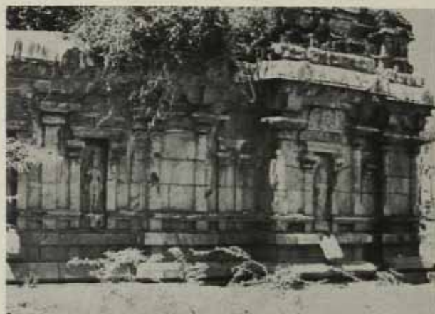
Pl 399 Kandalisvarar temple—North wall
