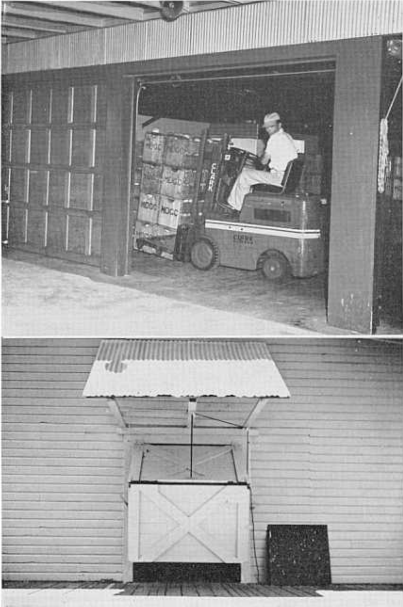
Fig. 16.—Above: Garage-type overhead doors used on the outside walls of degreening rooms. Note (top right) that canvas curtains are used for the interior walls. Below: A very simple and inexpensive home-made version.
