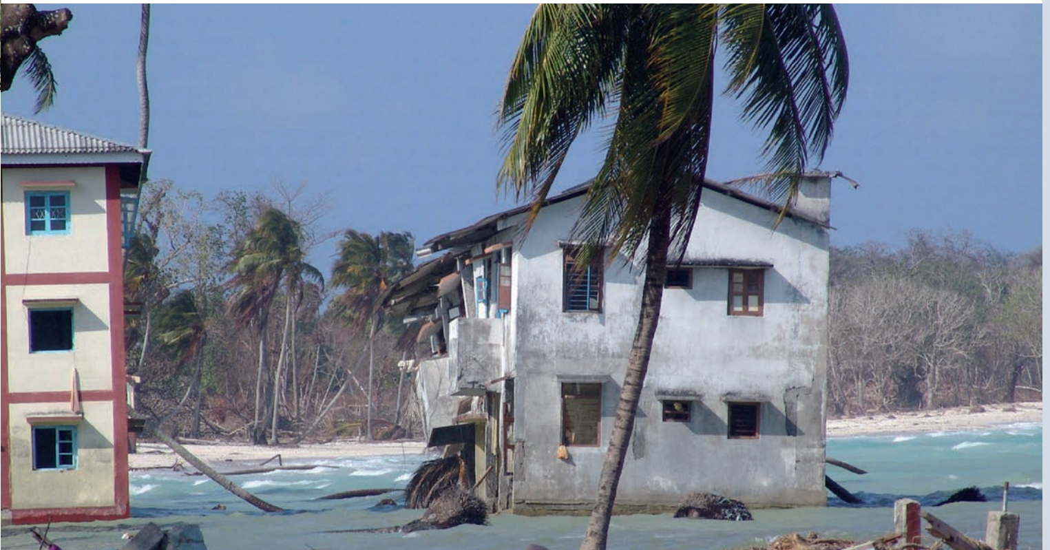
The 26 December 2004 earthquake resulted in 1.2 m of land subsidence in the Car Nicobar, Nicobar Islands, India, leaving houses that were once above sea level now permanently submerged. Photo courtesy of ICMAM, Chennai, DOD, India.
