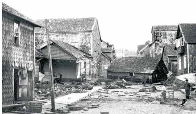
Damage caused by the 22 May 1960 Chilean tsunami. Photo courtesy of Ilustre Municipalidad de Maullin, USGS Circular 1187.
