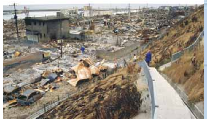
Massive destruction in the town of Aonae on Okushiri Island, Japan caused by the regional tsunami of 12 July 1993. Photo courtesy of Dr. Eddie Bernard, NOAA PMEL
