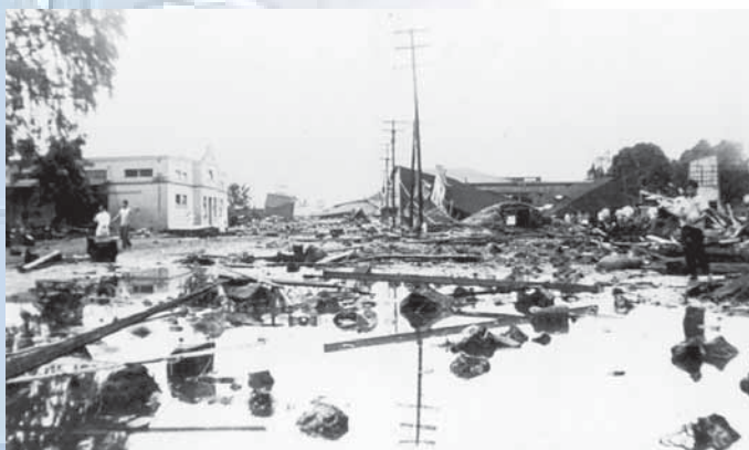
Destruction along the waterfront of Hilo, Hawaii from the Pacific-wide tsunami generated off the coast of Unimak Island, Aleutian Island, USA on 1 April 1946.
