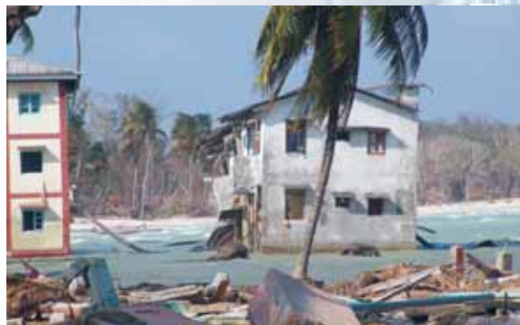
The 26 December 2004 earthquake resulted in 1.2 m of land subsidence in the Car Nicobar, Nicobar Islands, India leaving houses that were once above sea level now permanently submerged. Photo courtesy of ICMAM, Chennai, DOD, India.
