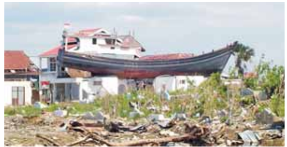
Runup can often be inferred from the vertical extent of dead vegetation, from debris normally found at ground level that are observed stuck on electric wires, in trees, or at other heights, and from water line marks left on building walls. In extreme cases, cars, boats, and other heavy objects have been lifted and deposited atop buildings. Banda Aceh, Indonesia, 26 December 2004. Photo courtesy of C. Courtney, Tetra Tech EMI.
