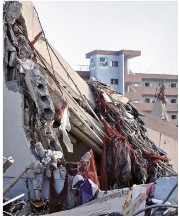
Tall reinforced concrete buildings served as vertical evacuation refuges during the 11 March 2011 Japan tsunami, saving many lives. Minami Sanriku, Japan. Photo courtesy of ITIC.
