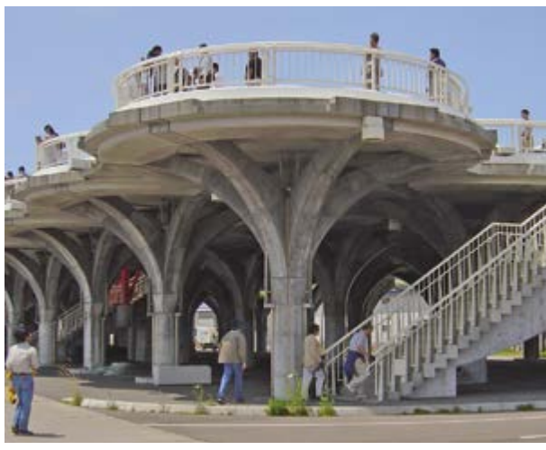
Elevated platform used for tsunami evacuation that also serves as a high-elevation scenic vista point for tourist. Okushiri Island, Japan. Photo courtesy of ITIC.
