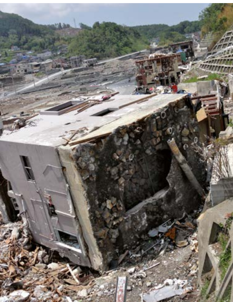
Tsunami flow depths exceeding 10 m and flow velocities over 6 m/s overturned and dragged 3-story buildings as much as 50 m during the 11 March 2011 Japan tsunami. Onagawa, Japan. Photo courtesy of ITIC.
