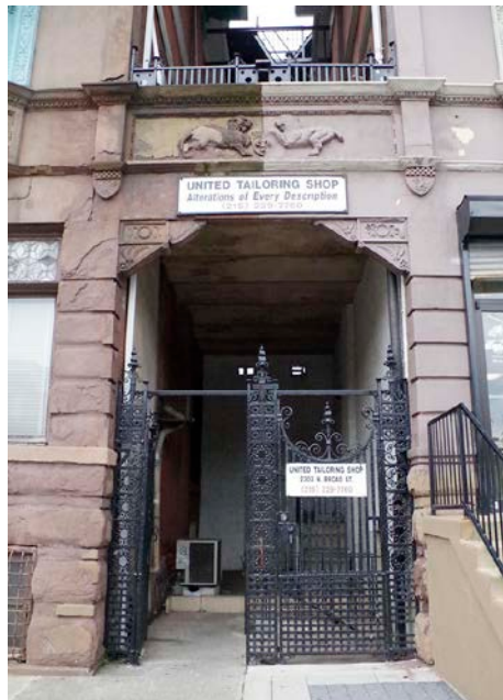
The connecting archway between the two buildings with decorative brownstone elements and an elaborate gate that is early if not original.
