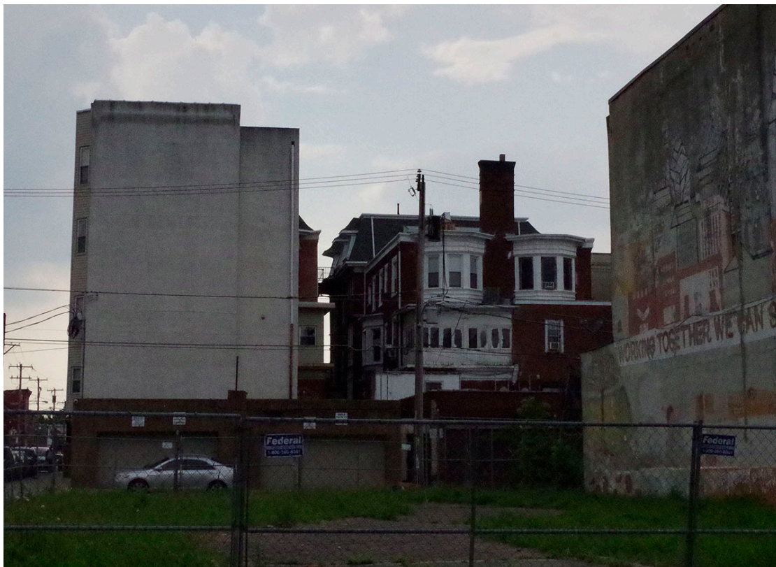
East elevation of both buildings at N. Watts Street. Photo: Author.
