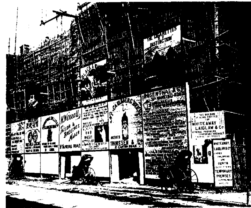
7.4 Advertising boardings on the building site of Shanghai's most luxurious department store, Whiteaway Laidlaw, show some of the variety of British business in the former treaty port.
