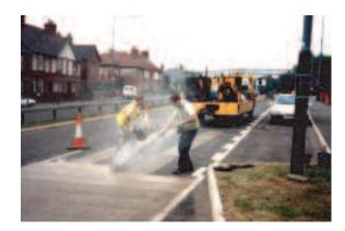
High-friction or 'anti-skid' surfacings are surfacings that make use of aggregates with better skid-resistance properties than normal, generally an artificial aggregate produced out of the "residue" from aluminium called calcined bauxite. In order for the aggregate to be retained on the surface with the high stresses expected, the binder needs to be stronger than can generally be achieved with conventional materials.
