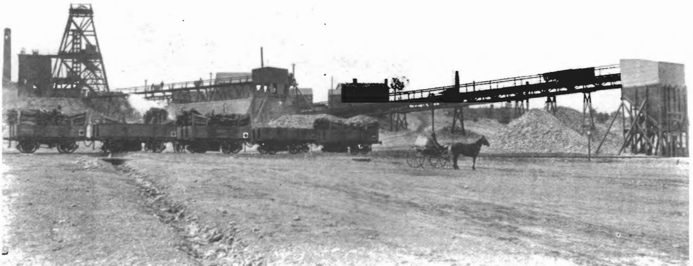
The Cobar Chesney Mine circa 1908, with standard gauge wagons loaded with firewood in the foreground. Behind, men push skips from the main shaft to a rock breaker, from which rakes of skips are rope-hauled to the ore bins on the right. Ore will be loaded in standard gauge hoppers for transport over The Peak branch line to the Great Cobar smelters. Courtesy Great Cobar Heritage Centre
