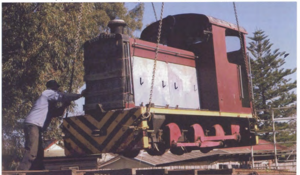
Kelly & Lewis 5957 is lowered onto the waiting truck in the grounds of Panania School on 15 July 2004.
