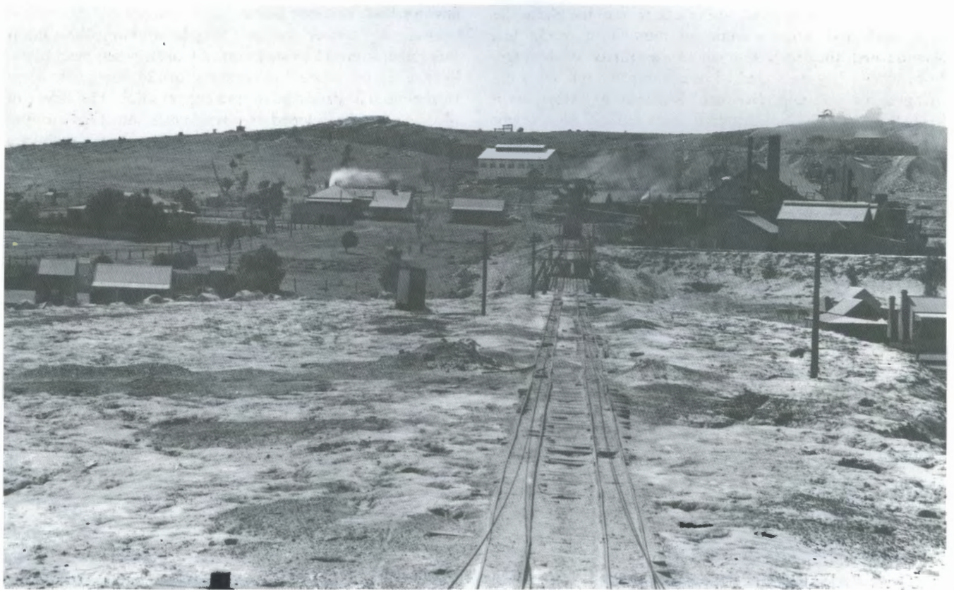
Cobar Gold Mine circa 1912, with the former haulage tramway to the waste disposal area being used to transfer ore to standard gauge hopper wagons on a siding off The Peak line below. A section of standard gauge track is visible on the right. The extensive treatment plant is centre right, with the main headframe further up Fort Bourke Hill. Courtesy Great Cobar Heritage Centre
