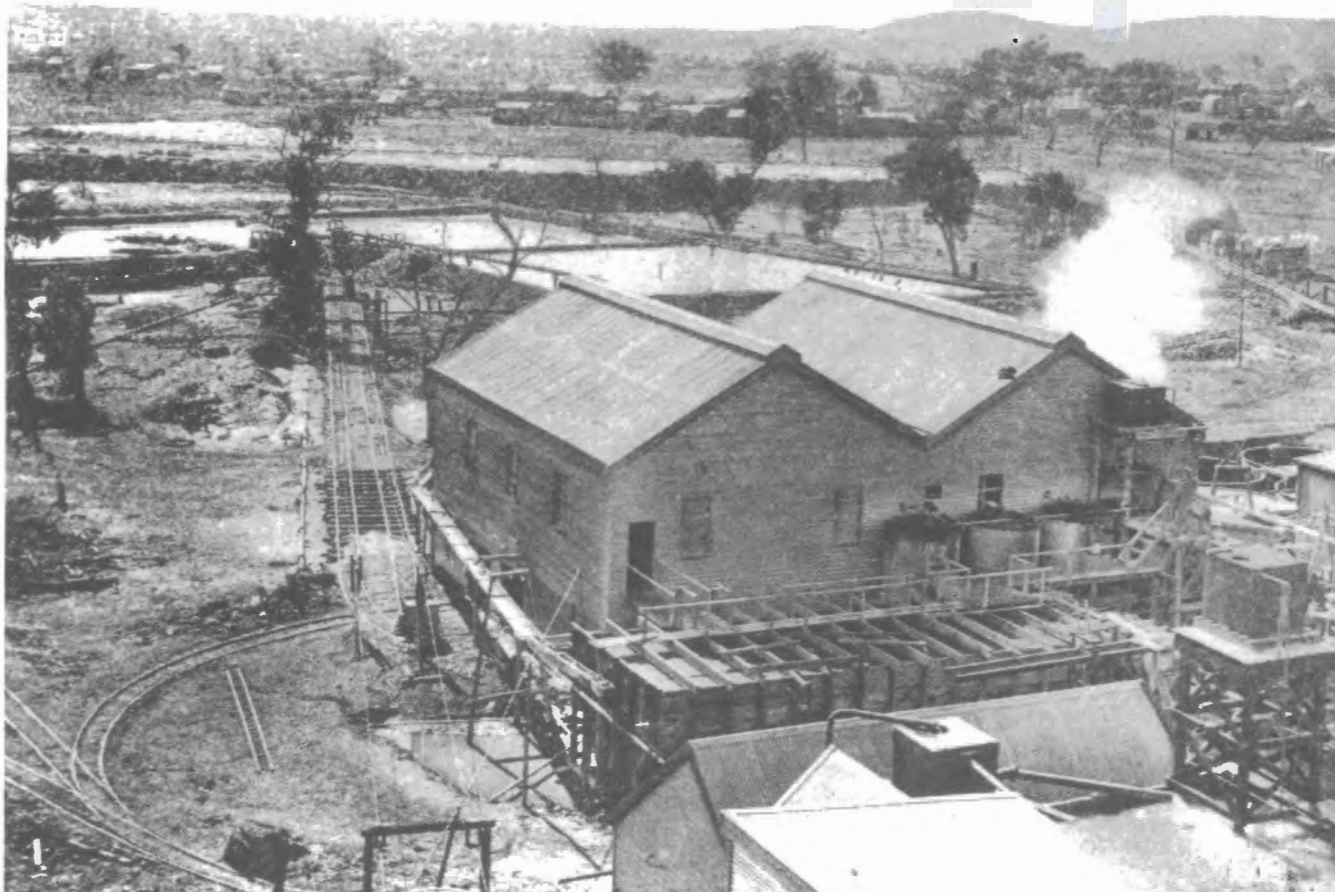
View of the Mt Boppy mine taken from the poppet head in 1905 looking over the building to the right of the previous photo to the village of Canbelago in the background. Note the rope-worked tramway to the tailing ponds and the various tracks in the foreground. The Sydney Mail, 12 July 1905
