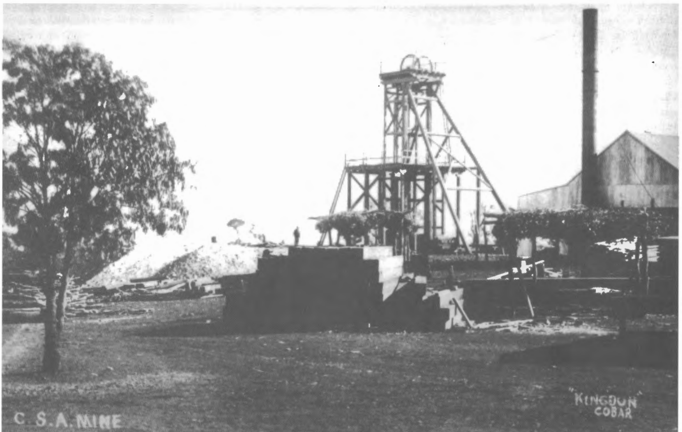
The CSA Mine in 1903, showing head frame and the winding house on the right.
