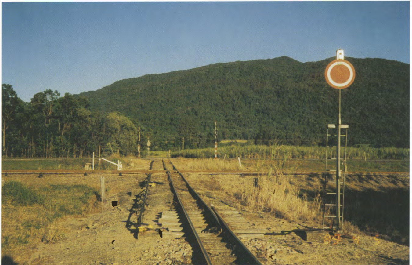
Looking east across the crossing of the QR in 1997 showing the catchpoint and signal arrangements. The Bruce Highway crossing is just past the rail crossing, and shortly beyond the line splits into northern and southern branches. Photo: Rod Milne
