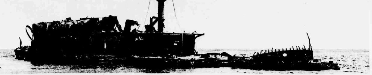
REMNANTS OF THE OLD TEXAS, TARGET USED IN FIRE CONTROL TESTS OF THE NEW NAVY. NOTE THE OLD MILITARY MAST, THOUGH RIDDLED BY SHELL FIRE, STILL IS STANDING, WHILE AT THE RIGHT THE BASE ONLY OF ONE OF THE NEW BASKET MASTS IS LEFT. Copyright E. Muller Jr. New York.
