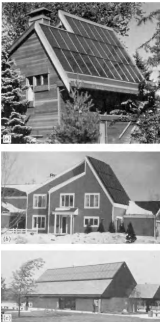
Figure 13.12.1 Three examples of solar heated buildings: (a, b) residences Madison, WI; (c) Wayside, Portage, WI.
