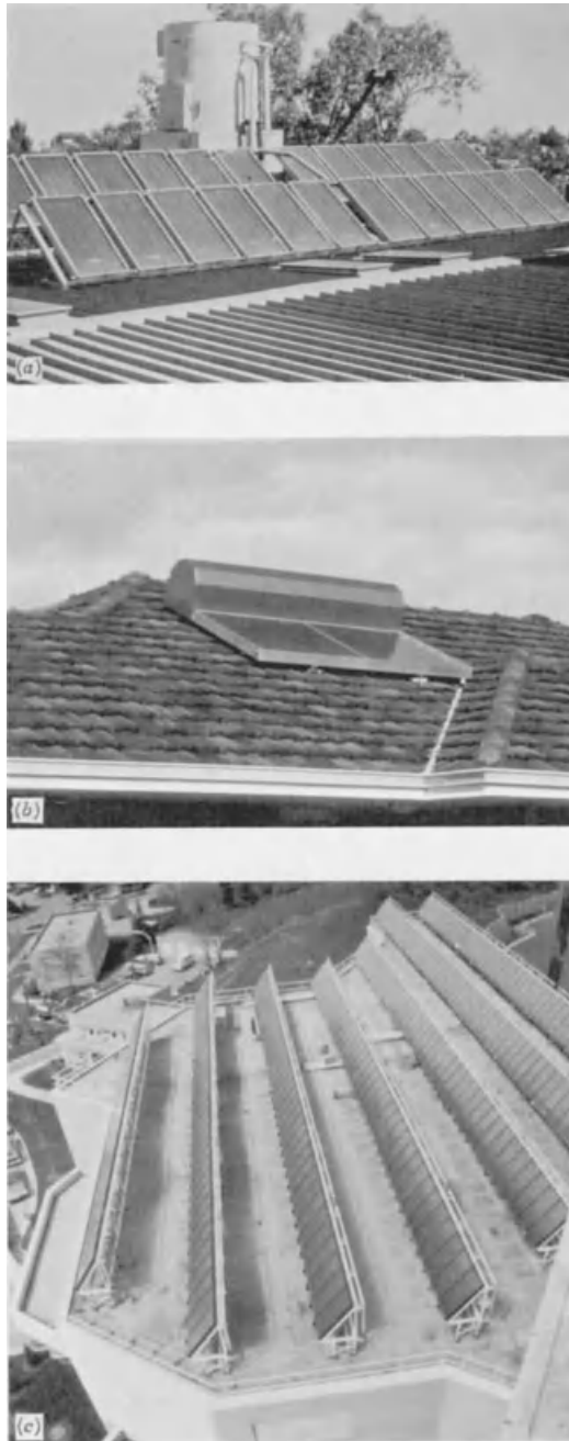
Figure 12.1.2 Solar water heaters. (a) Natural-circulation system on hostel, Griffith, Australia. Photo courtesy of CSIRO. (b) Domestic system, with coupled tank and collector, Perth, Australia. (c) Hospital service hot-water system, Madison, WI. Photo courtesy of Affiliated Engineers, Inc. (d) Collectors for a domestic system, Madison, WI.
