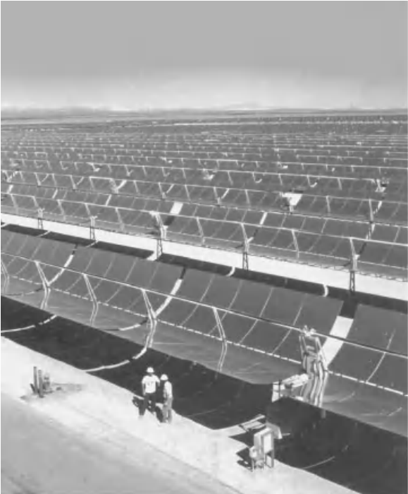
Figure 17.3.3 (a) SEGS collector fields.
