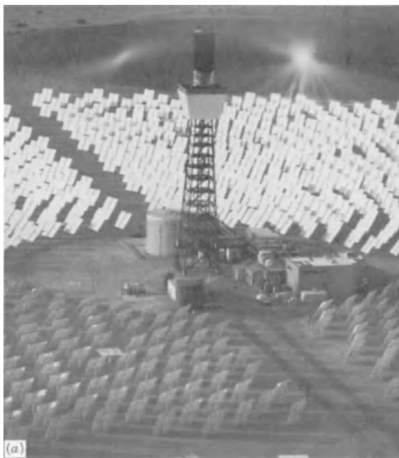
Figure 17.5.1 Solar One, at Barstow, CA. (a) Overall view of the heliostat field and receiver tower when system was not operating. (b) A heliostat. (c) The receiver, photographed from above, when in operation. Photographs courtesy of Sandia National Laboratories.
