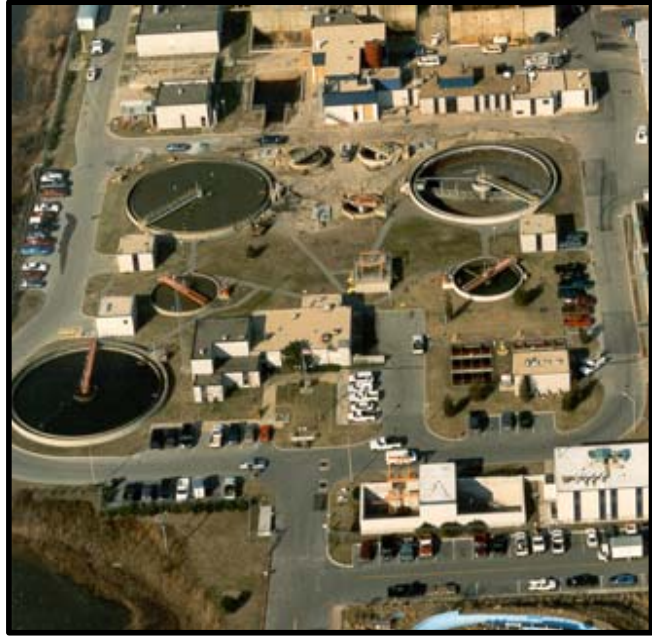
Wastewater Treatment Plant Facilities at 64 th Street
