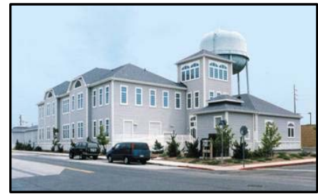
Water treatment plant at 15 th Street
