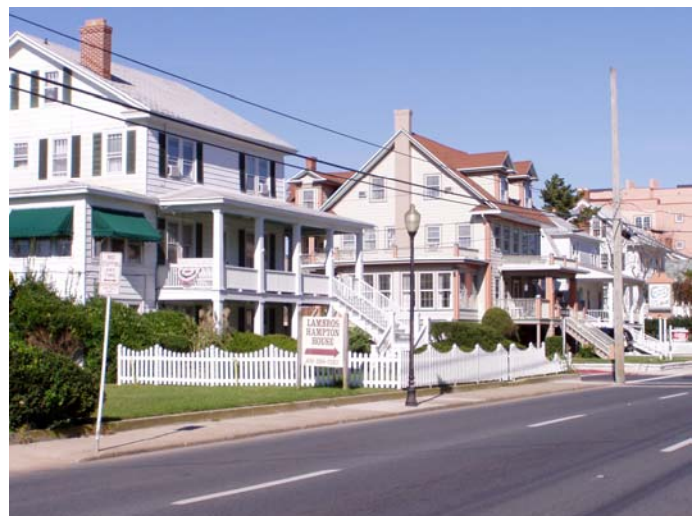
A number of Rooming Houses create old town charm and enhance the Baltimore Avenue Streetscape.
