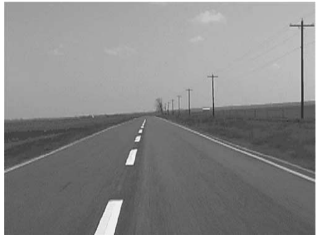
d. 8-inch line: 20-ft stripe, 20-ft gap
