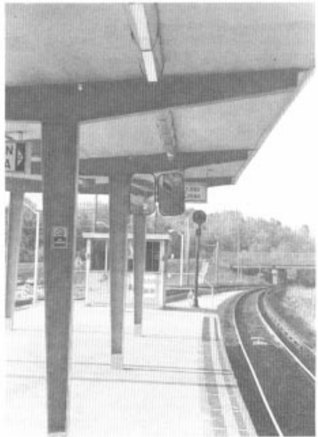
Figure 45. PATCO mirror installation.
