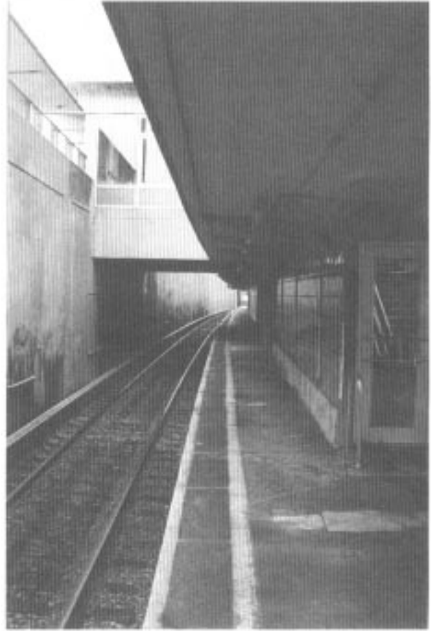
Figure 54. PATCO Haddonfield station curvature (westbound).
