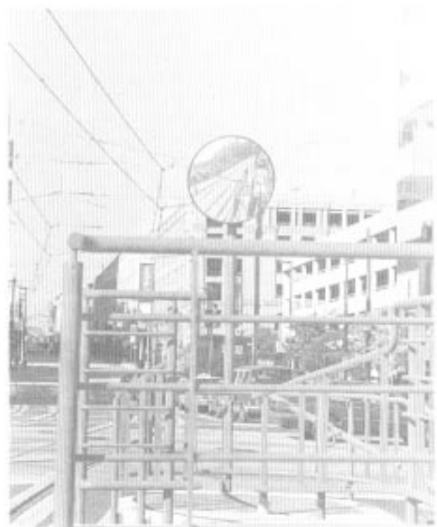
Figure 44. Baltimore MTA station mirror mounting.
