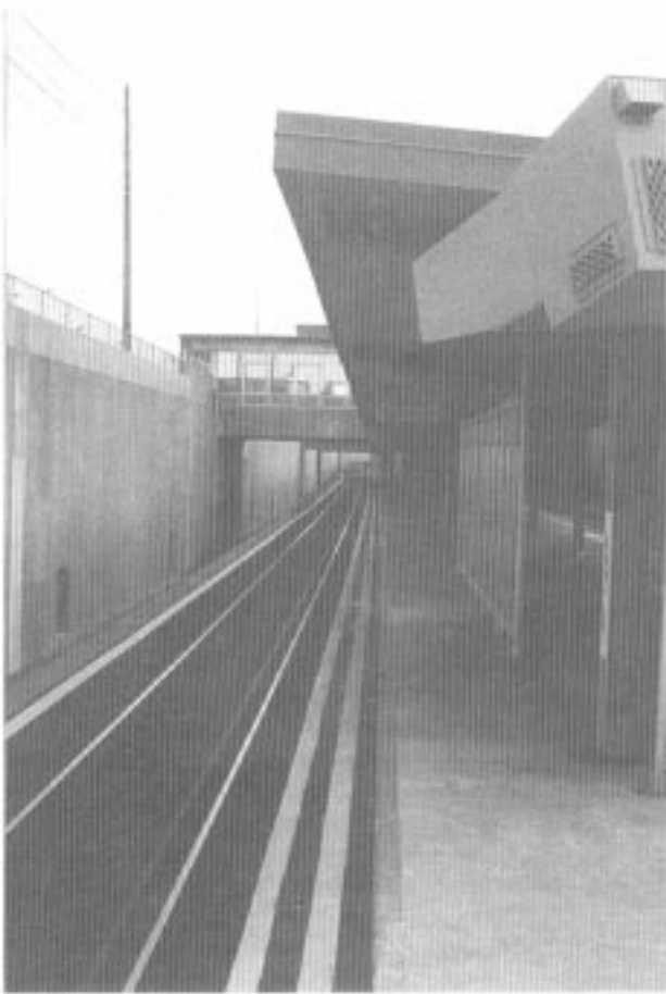
Figure 57. PATCO Haddonfield station monitor enclosure.
