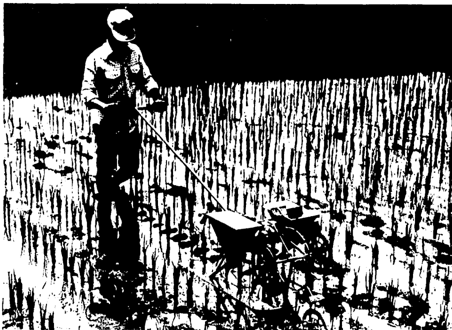
Fig. 8 Oscillating plunger applicator for prilled urea.
