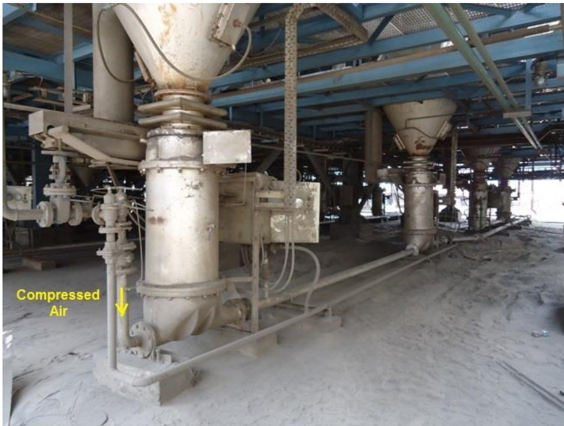
Typical Installation with Macawber's Ashveyor® System
