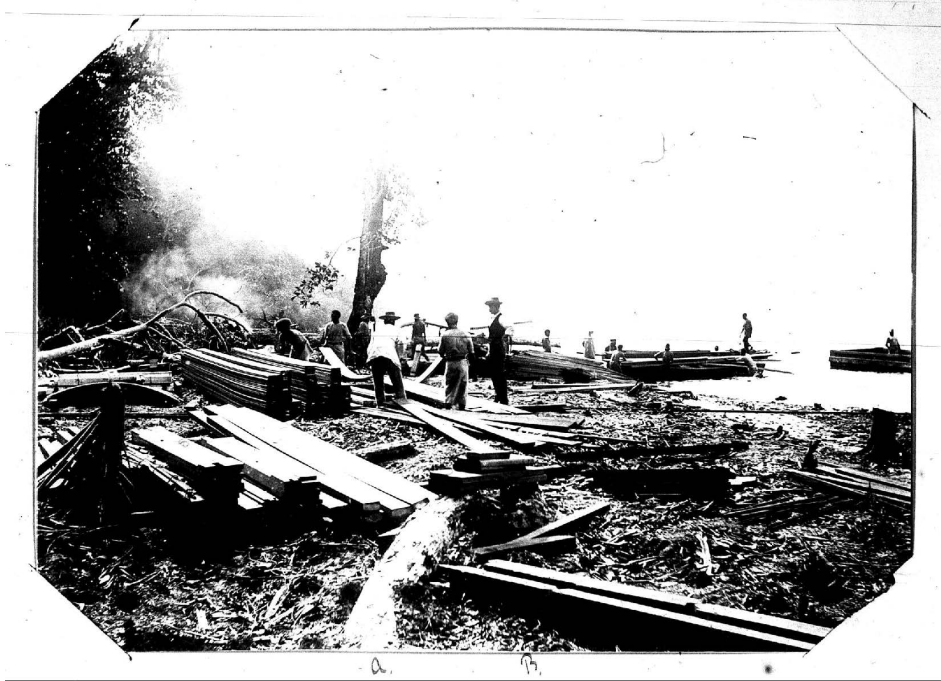
Figure 29. 'Unloading timber for Govt. Residence and Lock up at Tulagi. Photographed by Mr Lucas SS 'Titus'. a. Resident Commissioner. b. The Carpenter'.
