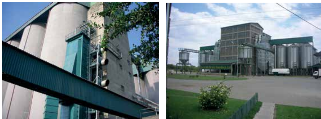
Figure 16. Lesiolo Grain Handlers' silos in Nakuru, Kenya
