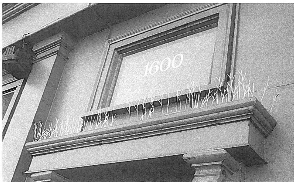
Figure 5. Anti-bird-roosting spikes on this heritage building protect patrons and the structure from soiling.
