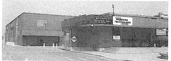
Level 4. A former bakery turned into a technology museum.
