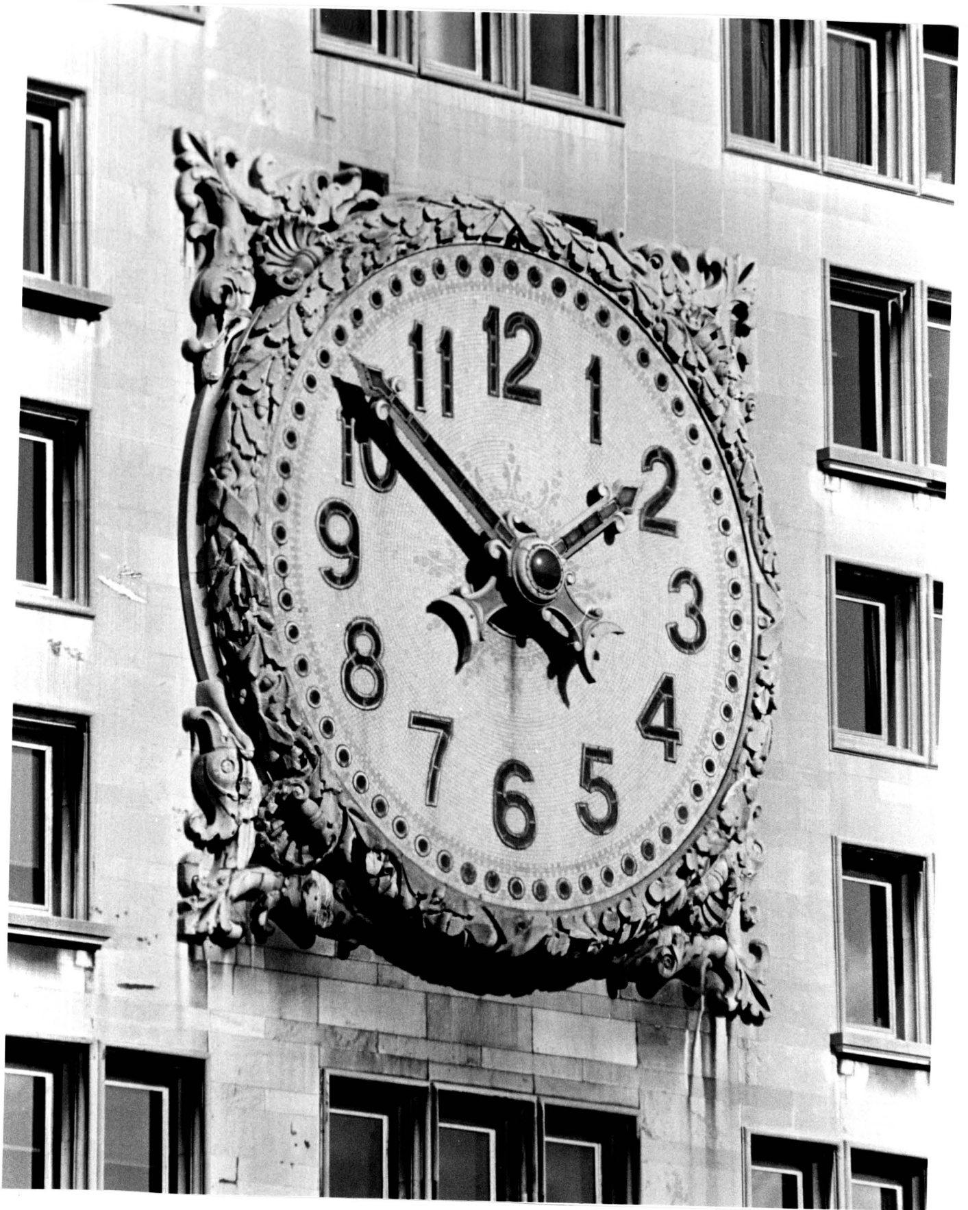
Plate 8. Clock face, south elevation.
