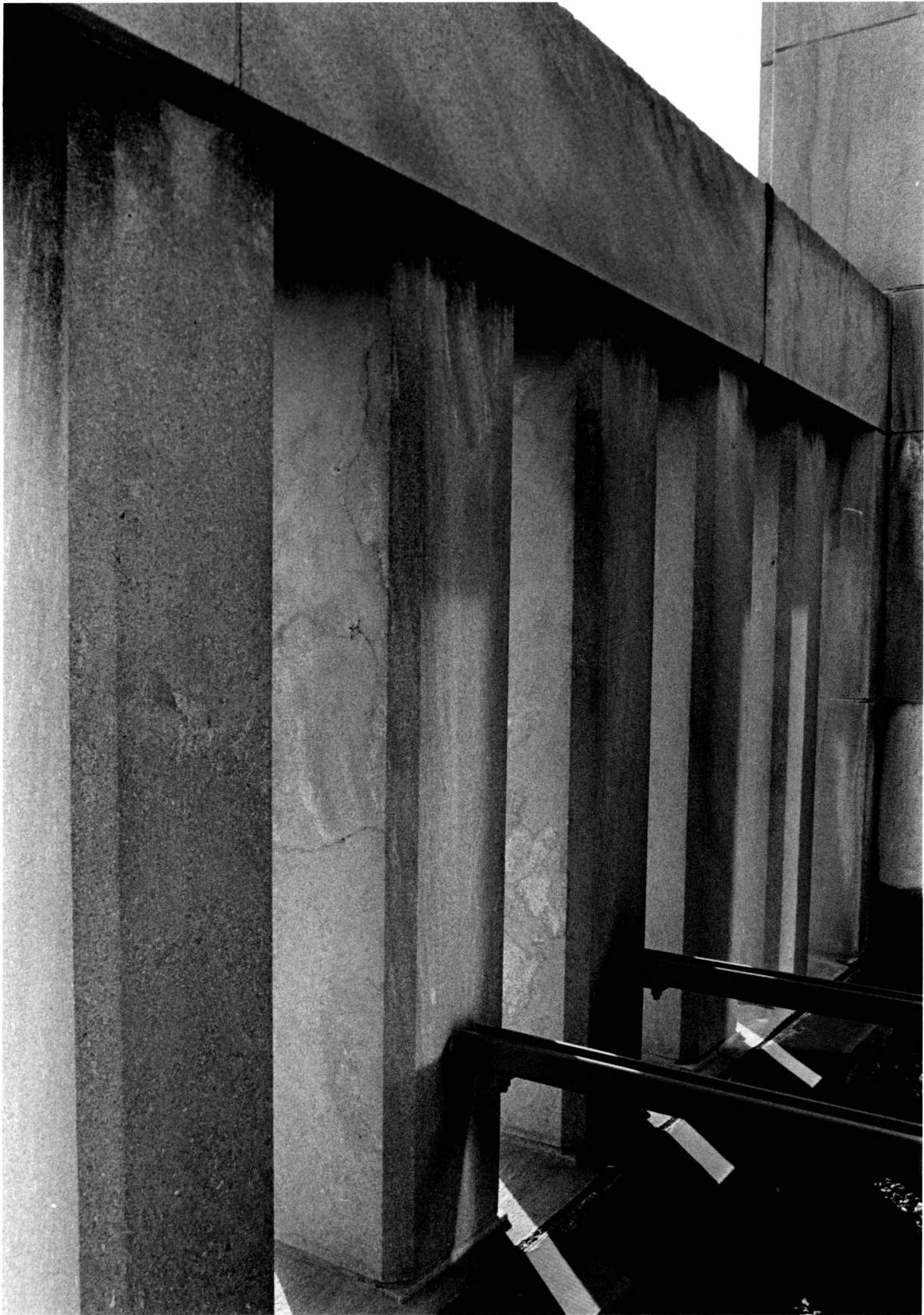
(Carl Forster) Plate 11. Chamfered balusters, arcade balustrade, thirty-first story, Metropolitan Life tower.
