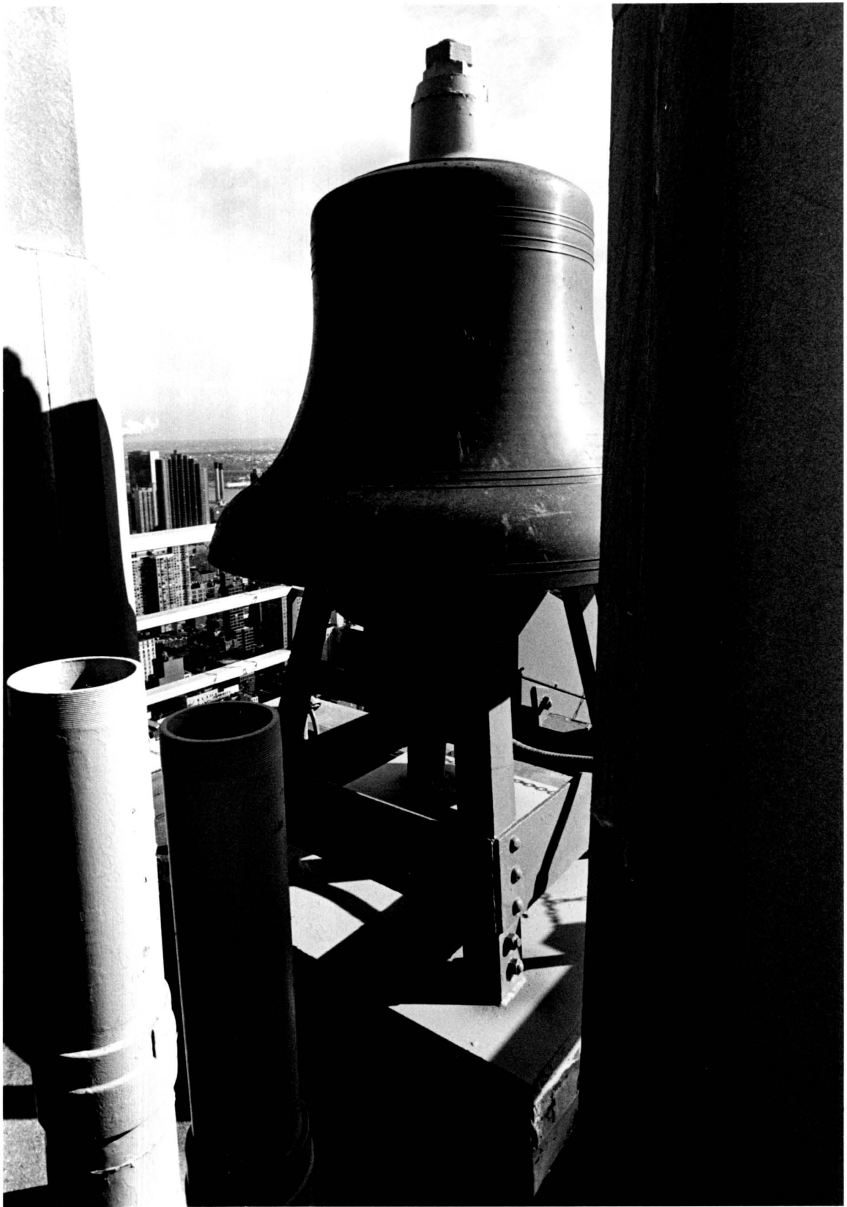
Plate 17. 3000 pound bell of the four bell chime, eastern elevation, the forty-sixth story. (Carl Forster)
