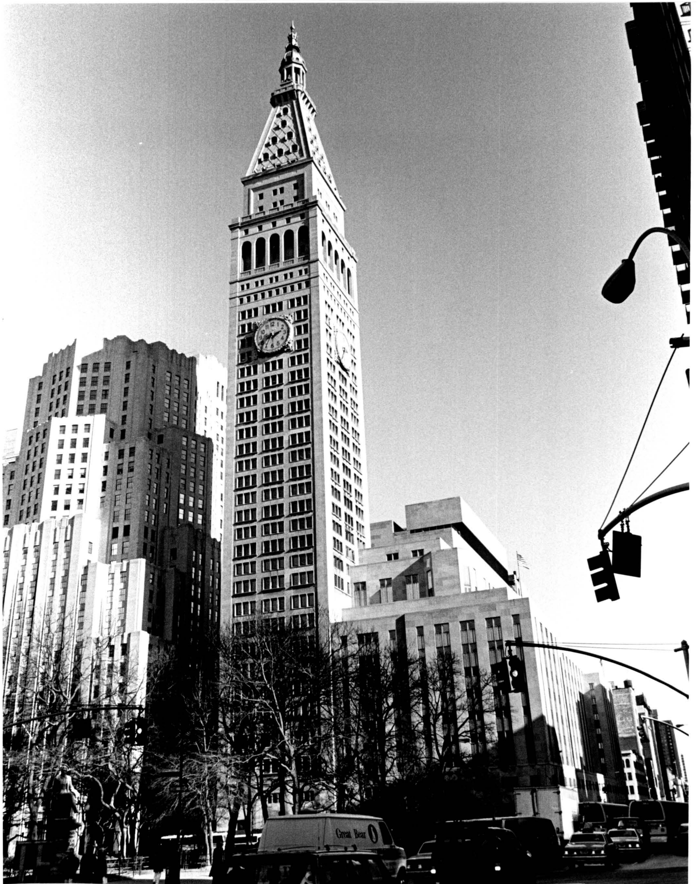
Plate 2. Metropolitan Life Insurance Company Tower, 1 Madison Avenue, built 1907-09. Renovated 1960-64. (Carl Forster)
