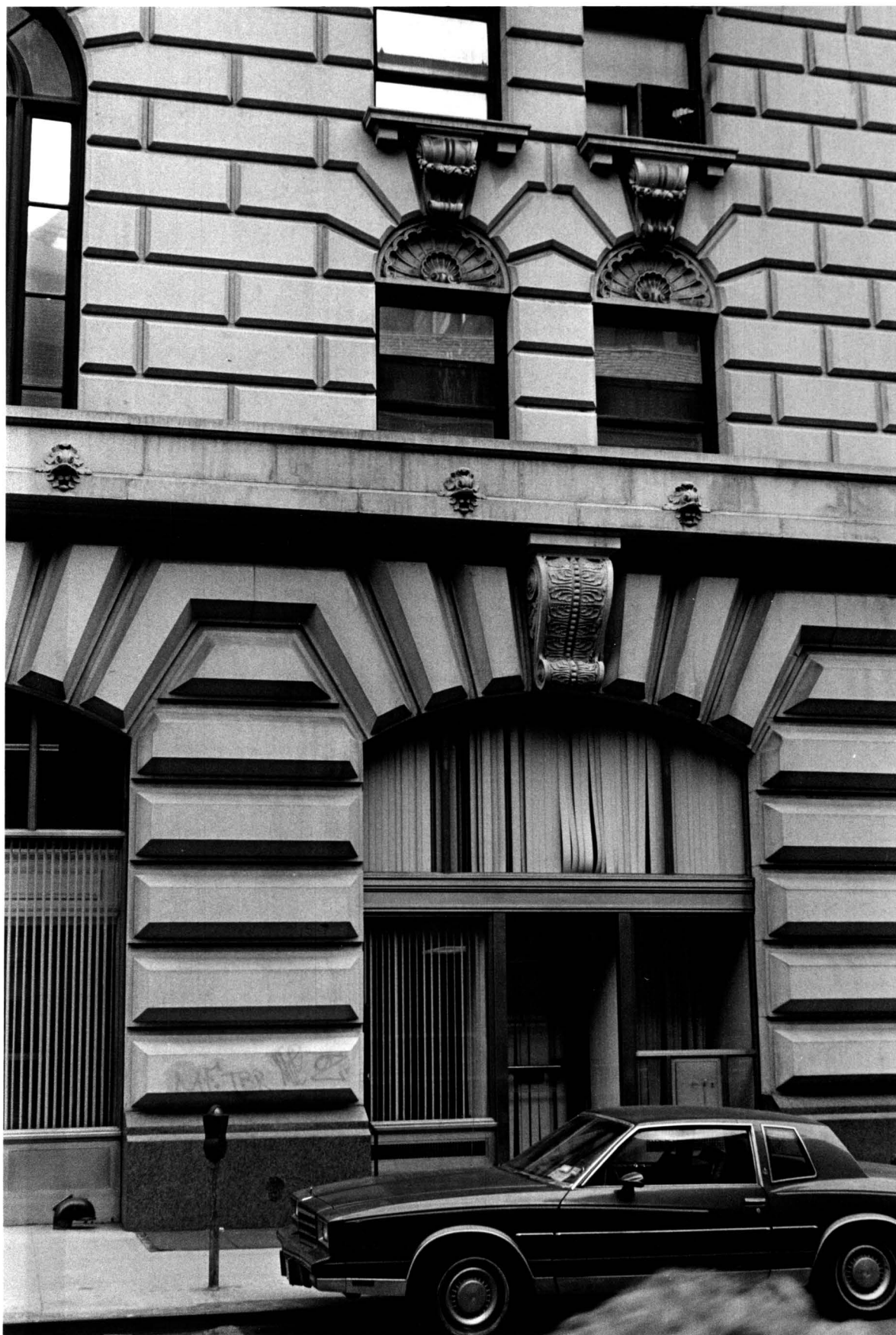
The Germania Life Insurance Company Building (now Guardian Life Building) Detail, ground and second stories
