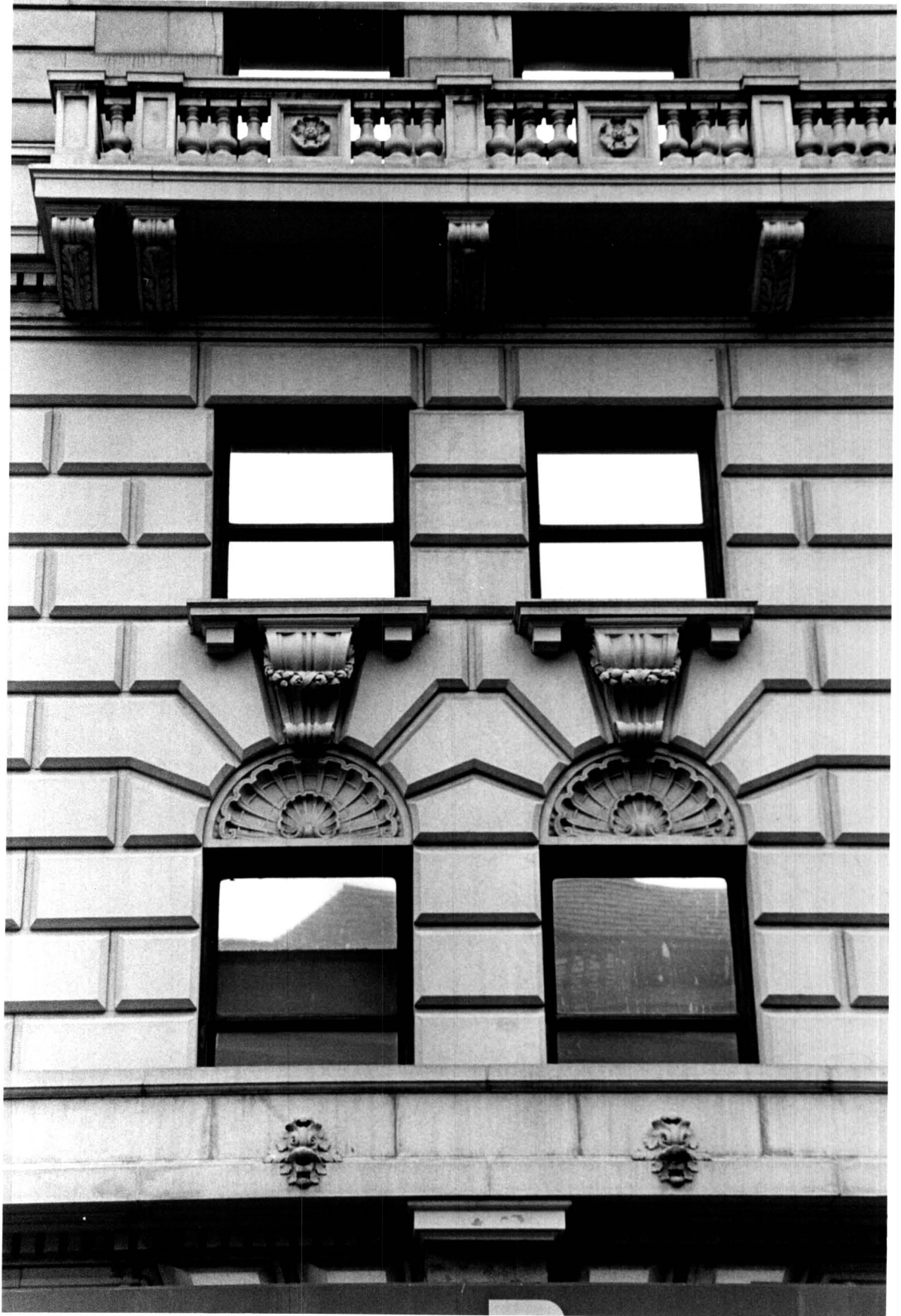
The Germania Life Insurance Company Building (now Guardian Life Building) Detail, second and third stories
