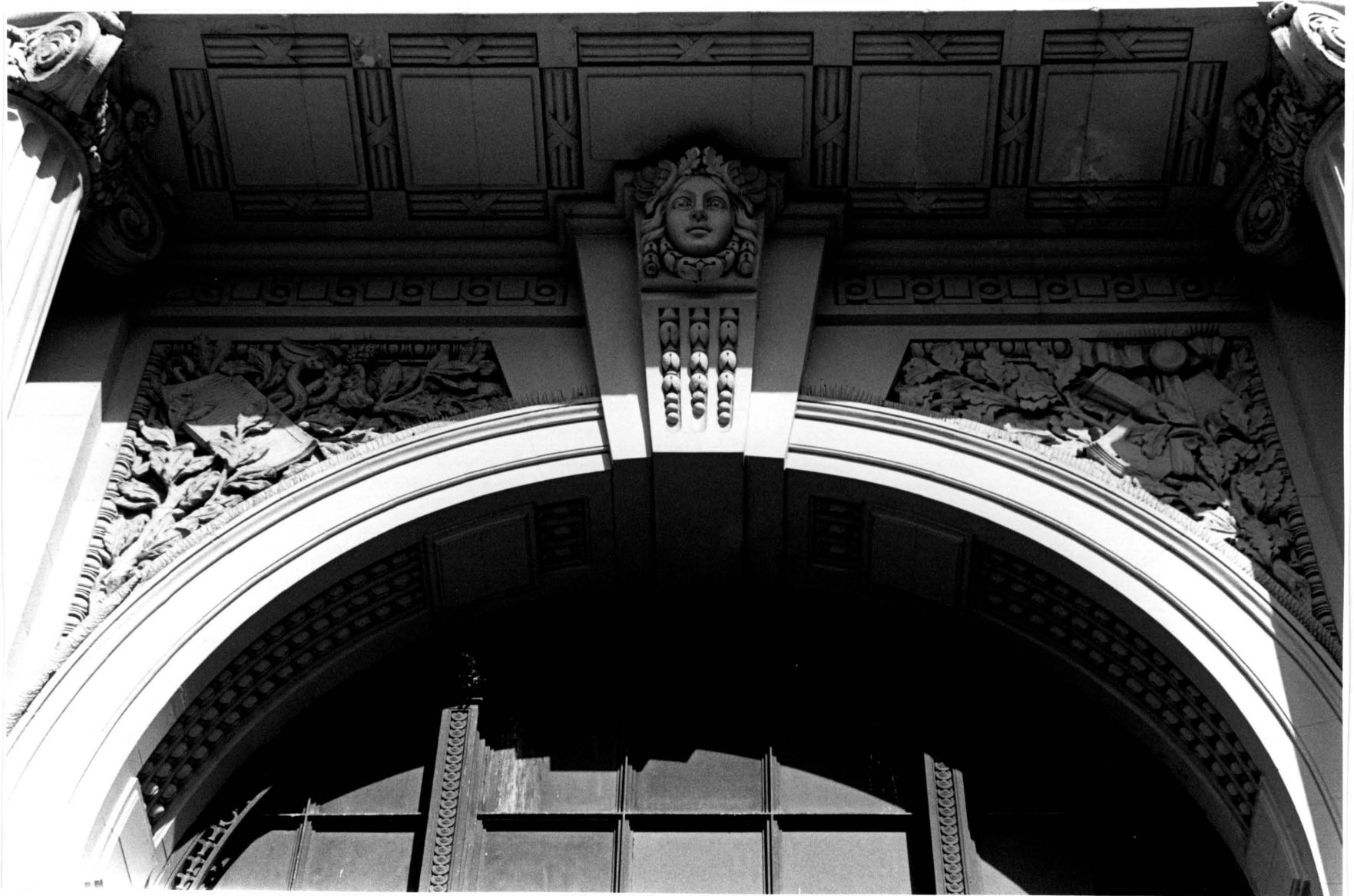
Manufacturers Hanover Bank Detail, Eighth Avenue facade, spandrels and keystone
