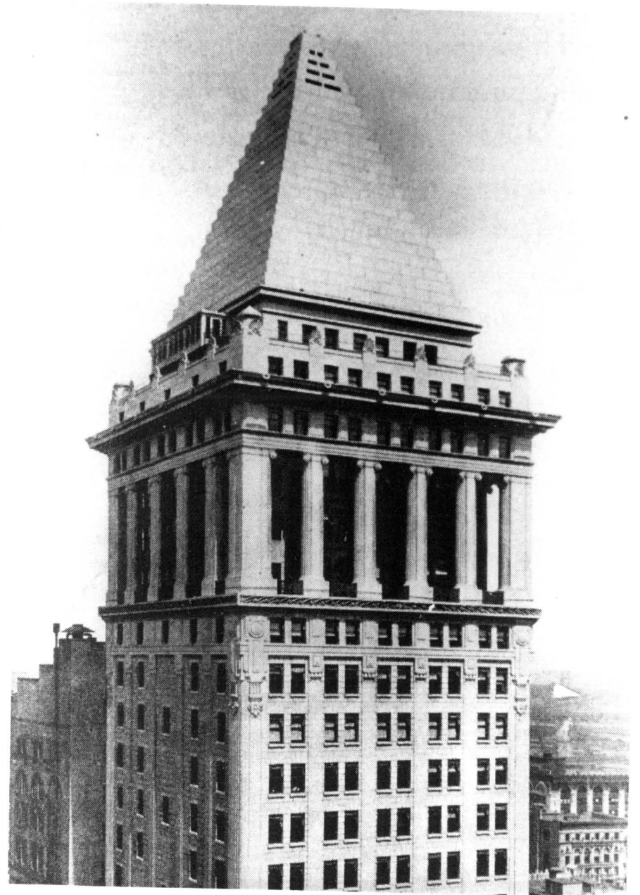
Historic Views showing the 14 Wall Street Tower (formerly Bankers Trust Building), c. 1912
