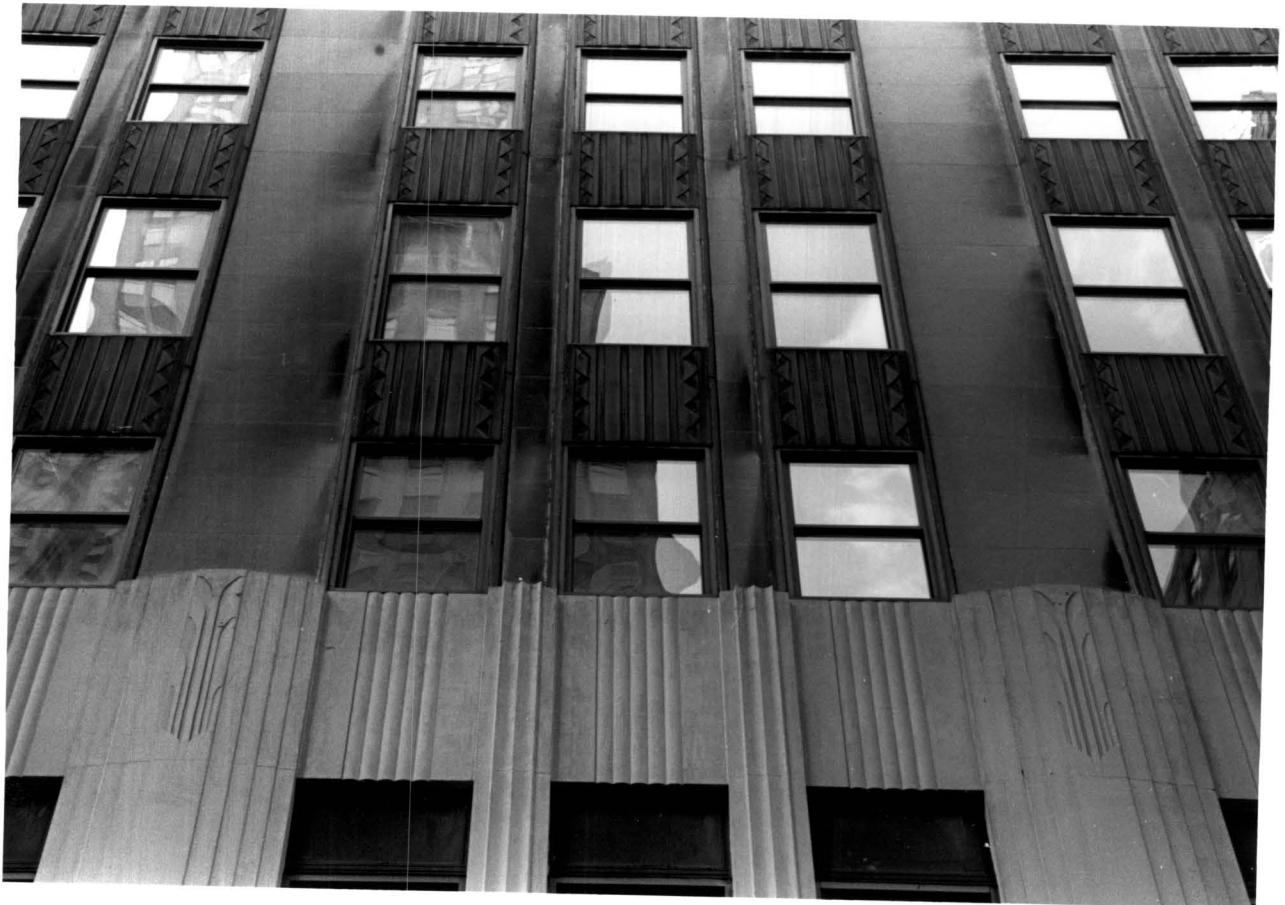
Details of the upper story articulation of the tower (top) and 1930s addition (bottom) on Nassau Street
