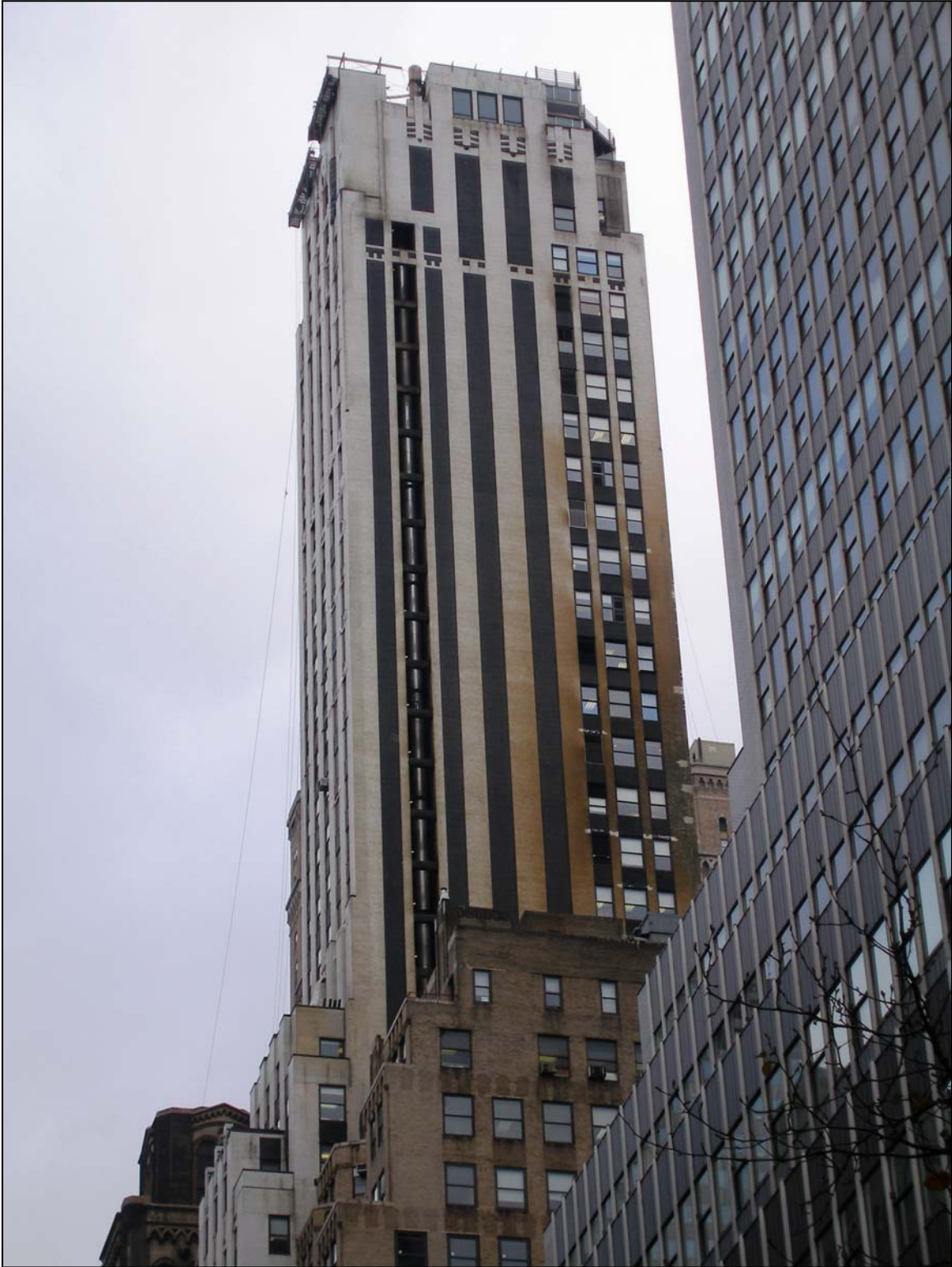
275 Madison Avenue South façade of upper tower Photo: Michael Caratzas, 2008
