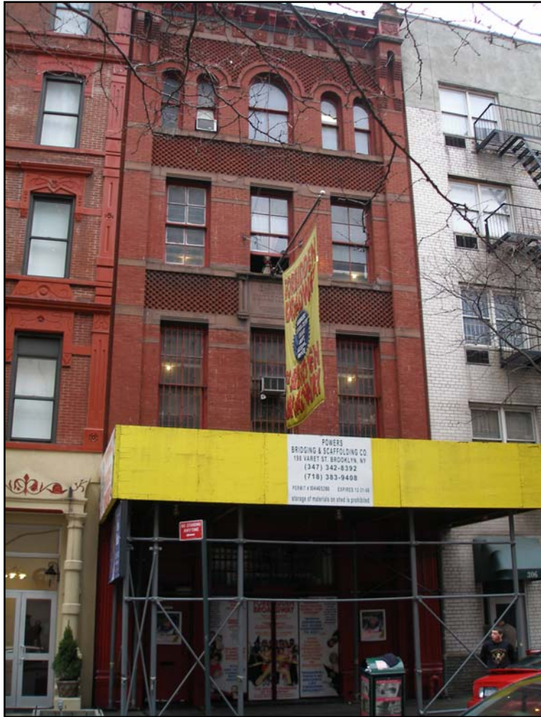
Fire Engine Company No. 54 304 West 47 th Street Photo by Theresa C. Noonan
