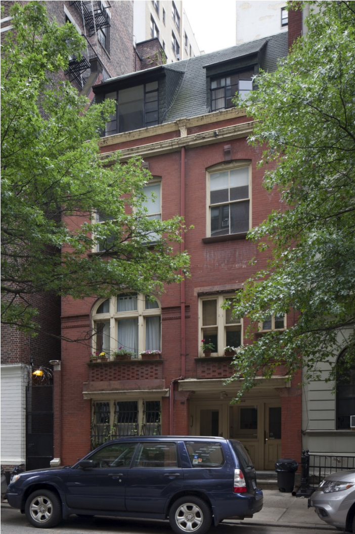
302 West 102 nd Street Ralph S. Townsend, 1884
