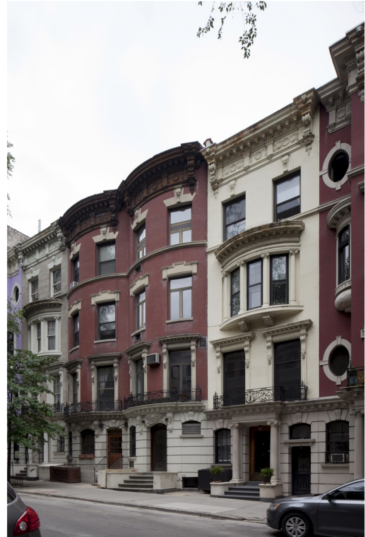
245 to 255 West 101 st Street Neville & Bagge, 1900-01
