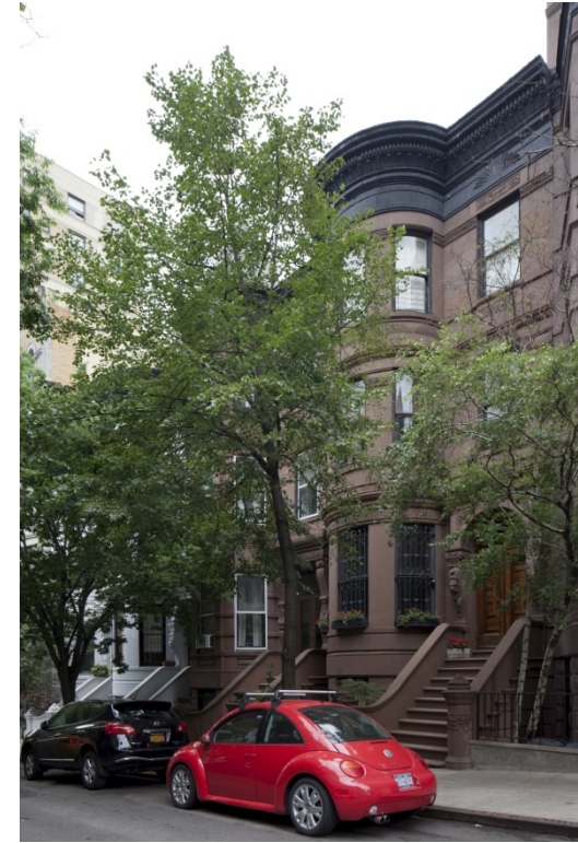
319 to 327 West 101 st Street Martin V. B. Ferdon, 1892
