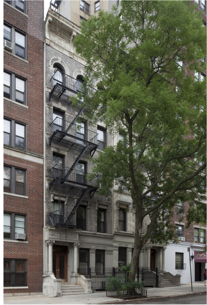
702 and 704 West End Avenue Neville & Bagge, 1895-96
