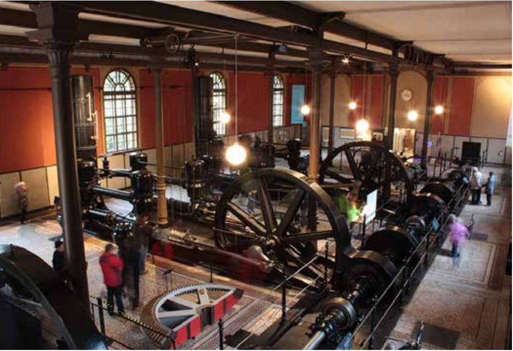
The double-acting piston pumps and air pressure vessels in the 1879 Hochablass water pumping station. (© Felix Hartmann, Wikimedia Commons)
