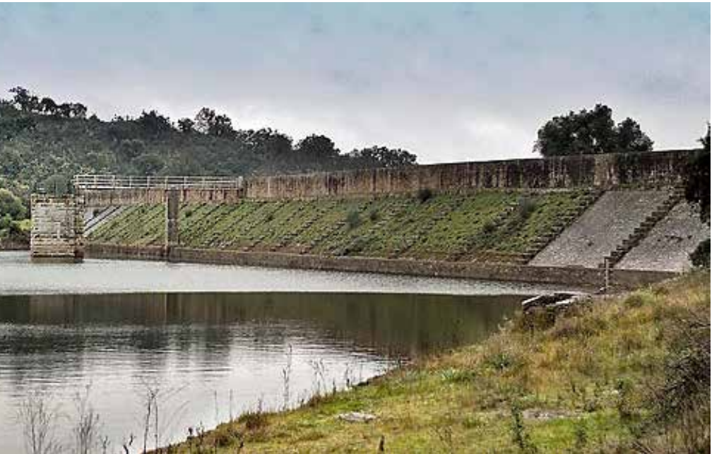
The Cornalvo gravity dam supplied water to the Roman city of Mérida in Spain. (© Charly Morlock, Wikipedia Commons)
