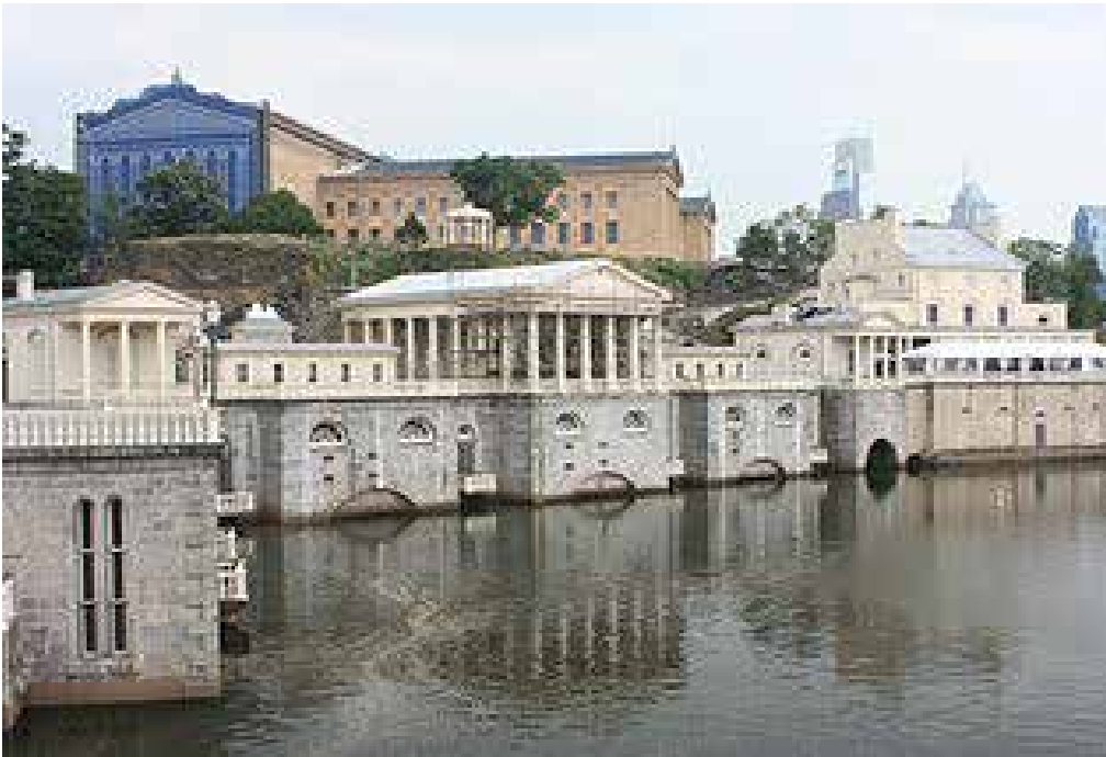
The Fairmount waterworks on the Schuylkill river in Philadelphia where waterwheels replaced beam engines to work the lift pumps. (© Ben Franske, Creative Commons)
