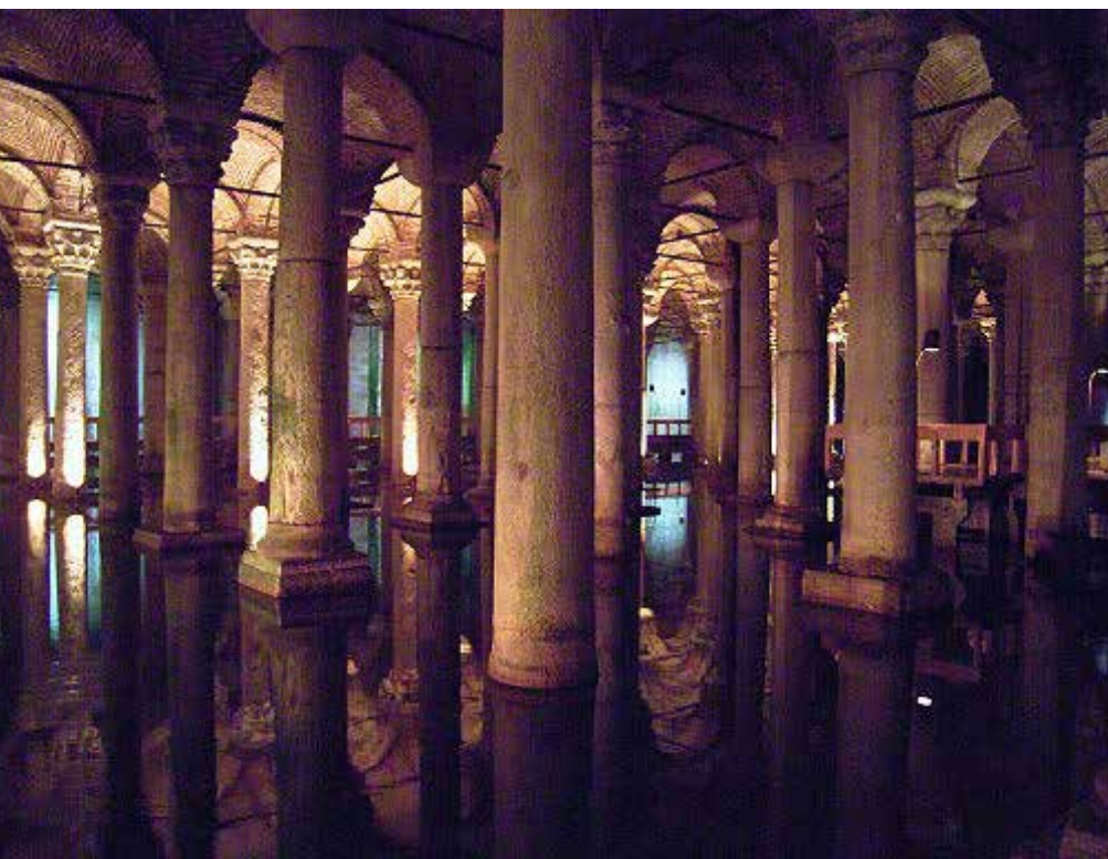
Recycled columns support the vaults of the Yerebatan cistern in Istanbul. Water was brought 19 km through channels incorporating two Roman aqueducts. (© Robert Raderschatt, Creative Commons)
