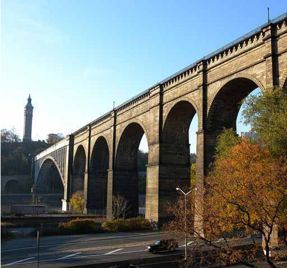
The 1837–48 High Bridge entering Manhattan. Most of the masonry arches were replaced by the 1927 steel arch. (© Jim Henderson, Wikimedia Commons)
