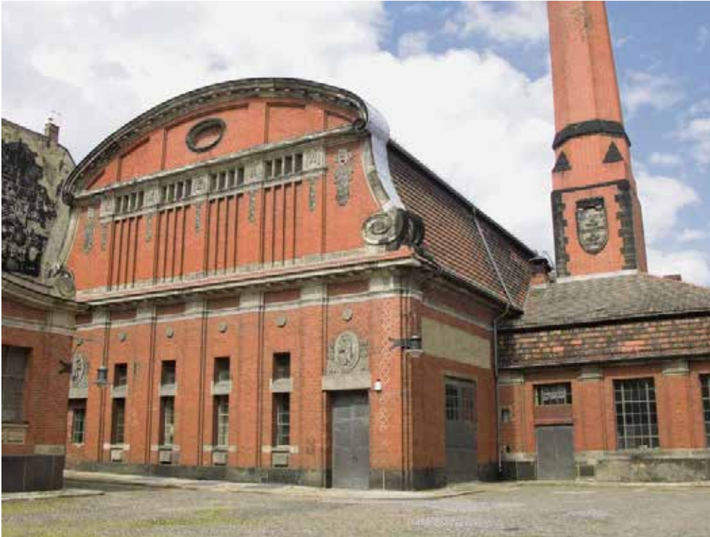
The Berlin sewage pumping station Radialsystem IX in Berlin. (Creative Commons)
