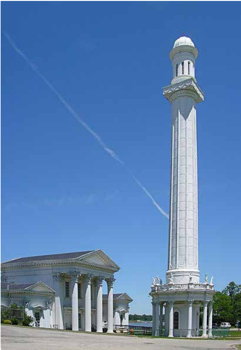
The Greek Revival pumping station and its cast-iron standpipe tower in Louisville, USA. The waterworks was built in 1860 by public subscription following a damaging fire and a cholera epidemic. (Creative Commons)
