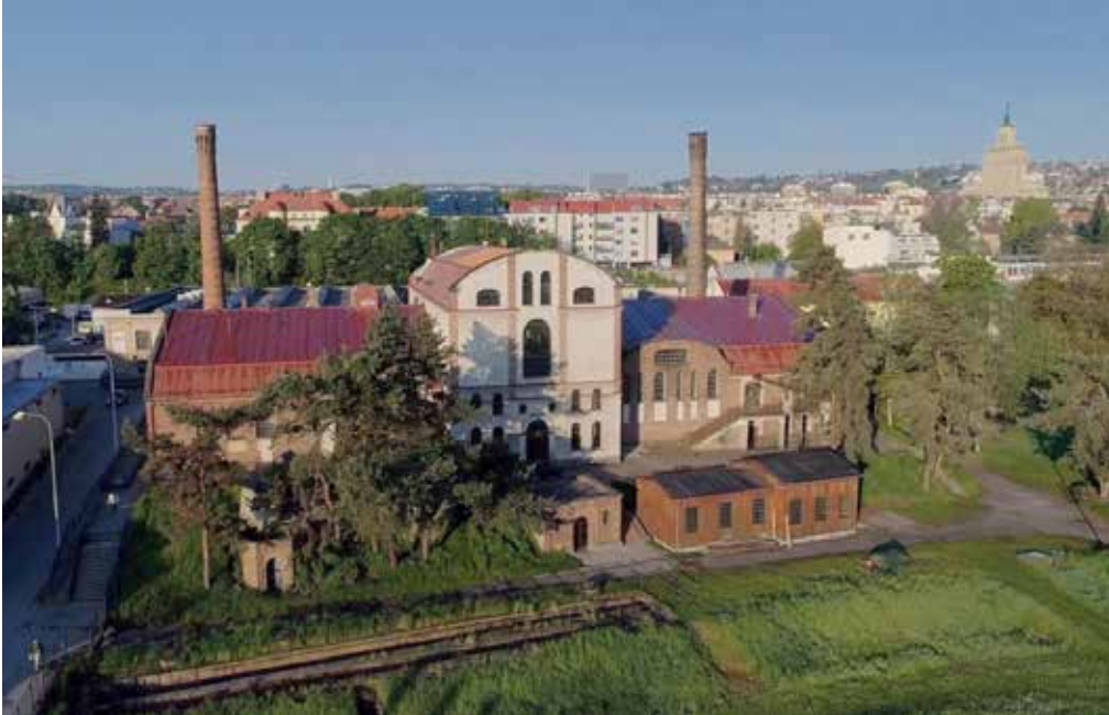
The complex of sewage pumping station and treatment plant at Prague-Bubeneč. (Wikipedia Commons)
