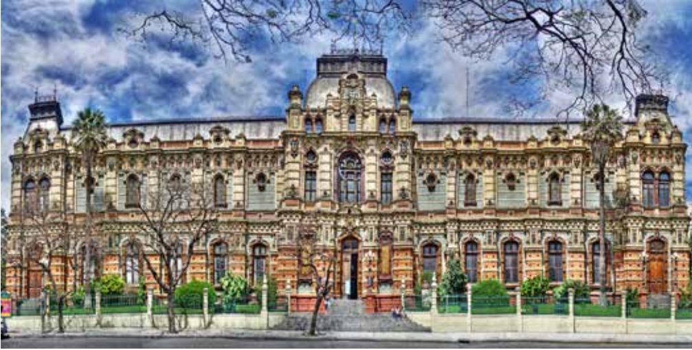
The glazed ceramic exterior of the Palacio de las Aguas Corrientes. (Wikipedia Commons)
