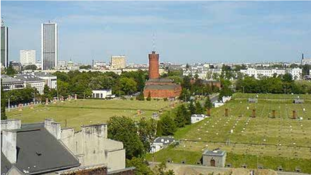
Filtry Lindleya (Lindley's filters) opened in 1886 to distribute filtered river water in Warsaw. Named after the prolific water engineer William Lindley, it includes a group of slow sand filters, covered reservoir, pumping station and water tower. (Creative Commons)
