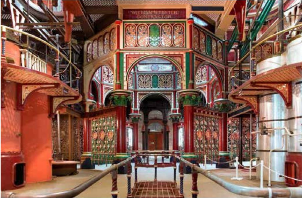
The restored interior of the 1865 Crossness sewage pumping station, London, had four single cylinder James Watt beam engines, converted to triple expansion operation in 1901 and 1902. (© Christine Matthews, Creative Commons)
