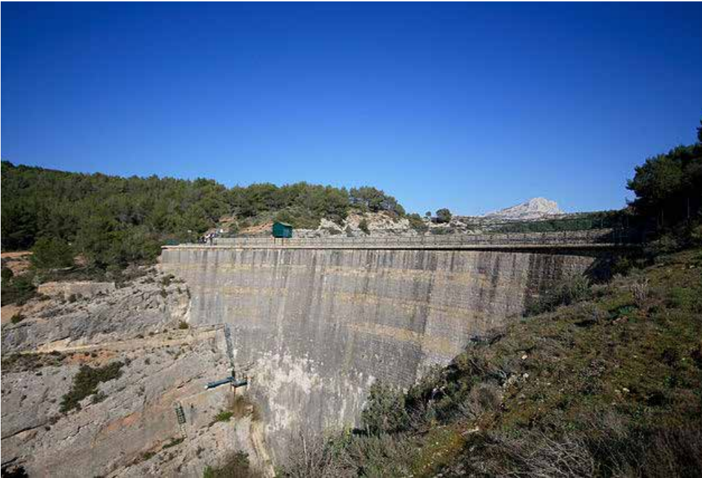
The Barrage Zola is an early masonry arch dam built to provide Aix-en-Provence with safe water following a cholera epidemic in the city. (Creative Commons)
