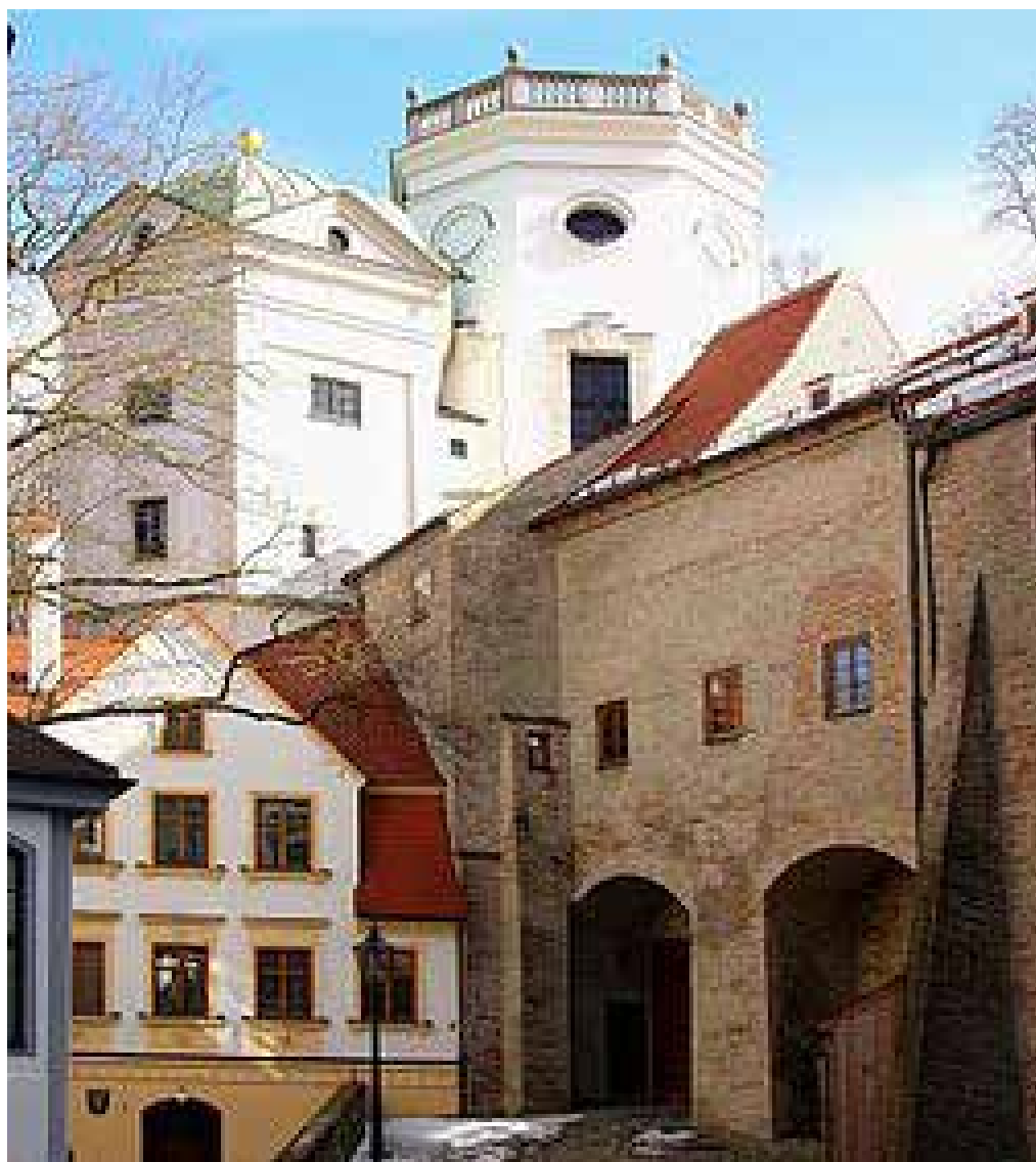
Piston pumps worked by waterwheels raised river water up to the Rotes Tor in Augsburg, Germany: Upper Brunnenmeisterhaus (left), Kleiner Wasserturm (middle) and Großer Wasserturm (right). (Creative Commons)
