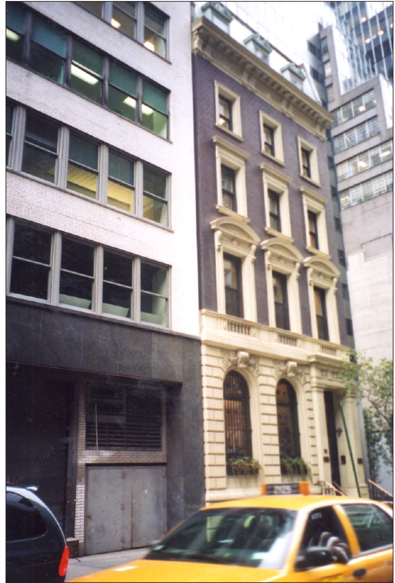
Townhouse at 39 East 51st Street 7
