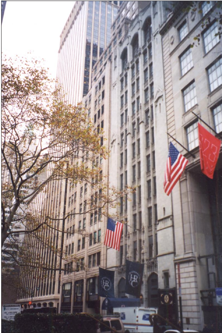
Former Grand Rapids Furniture Showroom and offices at 18-20 East 50th Street 6
