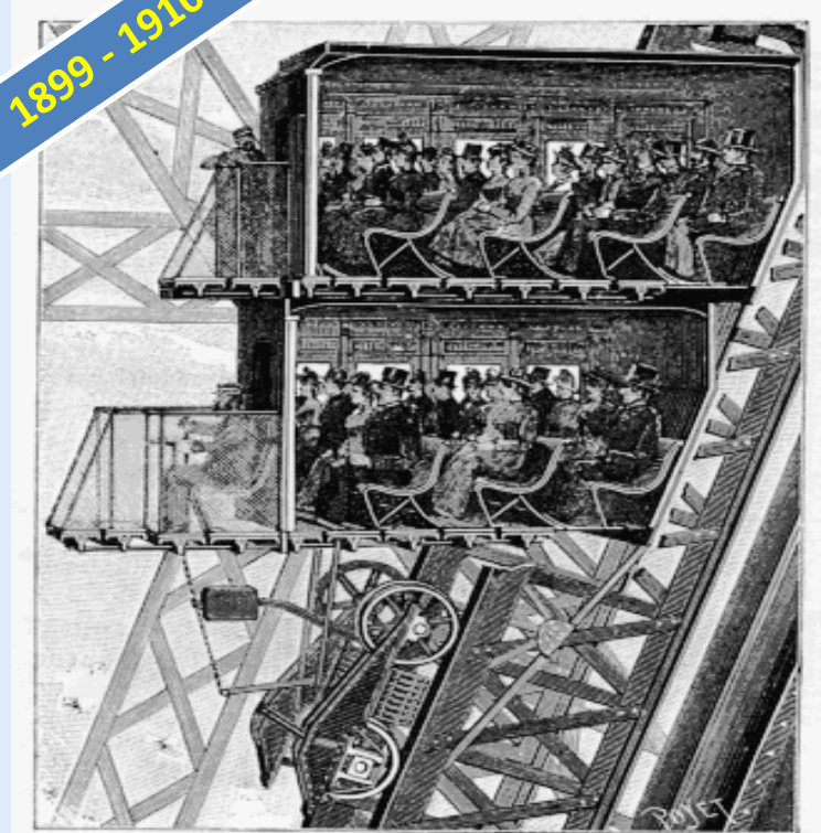
Figure 29.—Section through cabin of the Otis elevator. Note the pivoted floor-sections. As the car traveled, these floor-sections were leveled by the operator to compensate for the change of inclination; however, they were soon removed because they interfered with the loading and unloading of passengers. (From La Nature , May 4, 1889, vol. 17, p. 360.)
