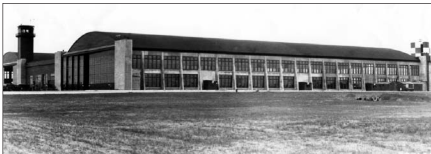
Hangars in 1943 at Great Falls Field (earlier, Gore Field), Montana, used to facilitate the transition through the base of Lend Lease aircraft bound for the Soviet Union.
