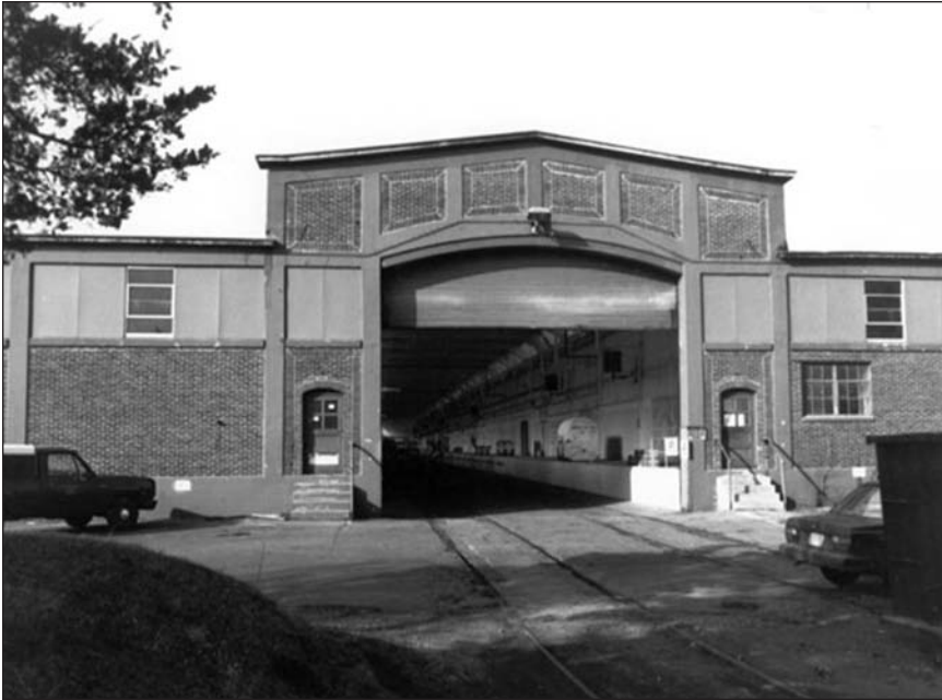
The oldest military building extant at Wright-Patterson AFB. Building 1 was constructed in 1917 as a warehouse for war materiel.
