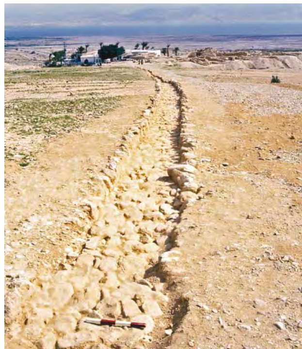
Fig. 40. Notice the construction of the aqueduct walls.
