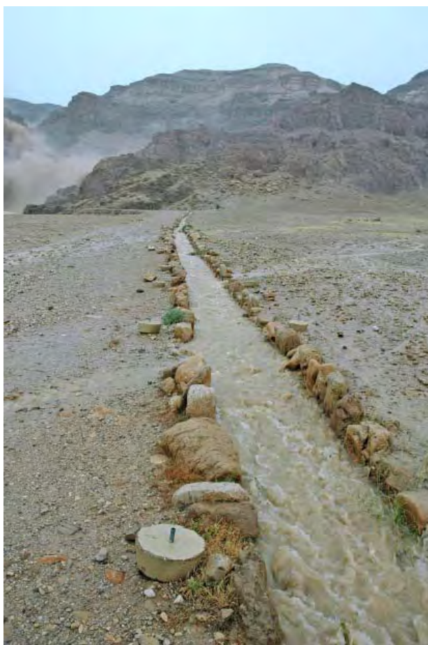
Fig. 41. Rainwater flowing in the aqueduct, Winter 2006 (courtesy of O. Gutfeld).
