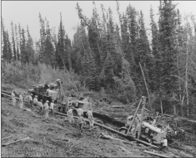
Figure 11. Haines-Fairbanks Pipeline construction. NARA.
