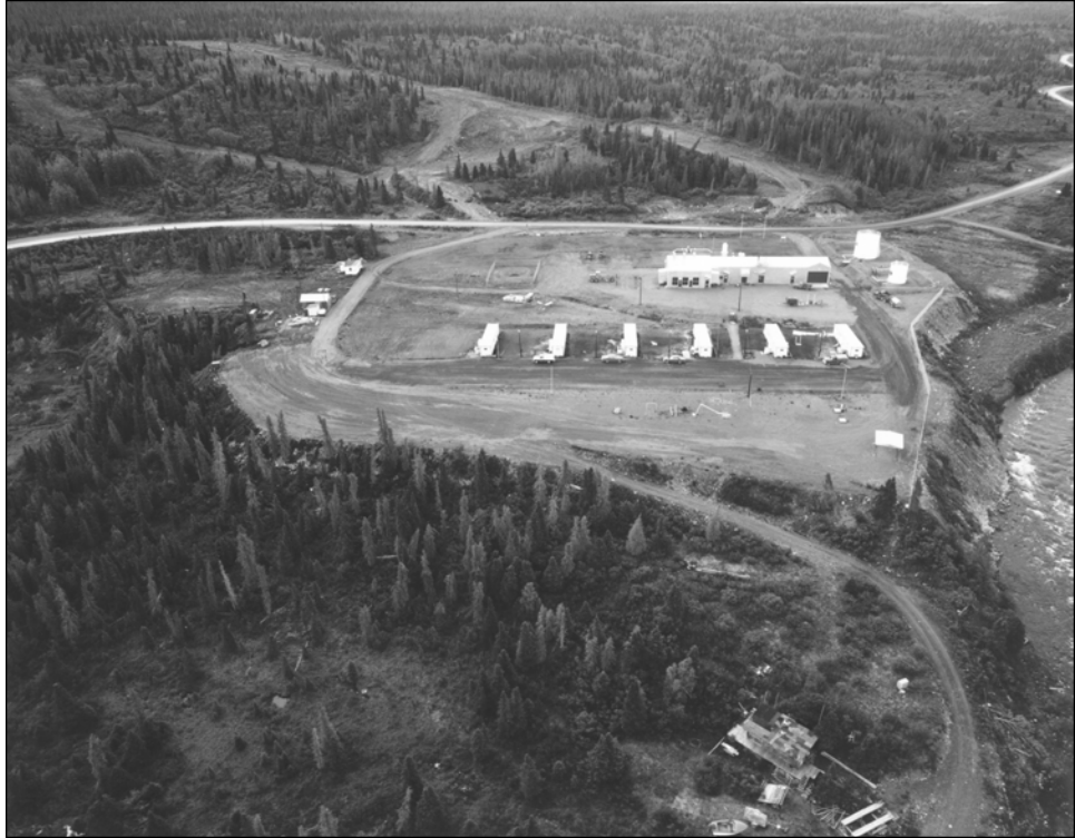
Figure 33. Blanchard River Pump Station. NARA.
