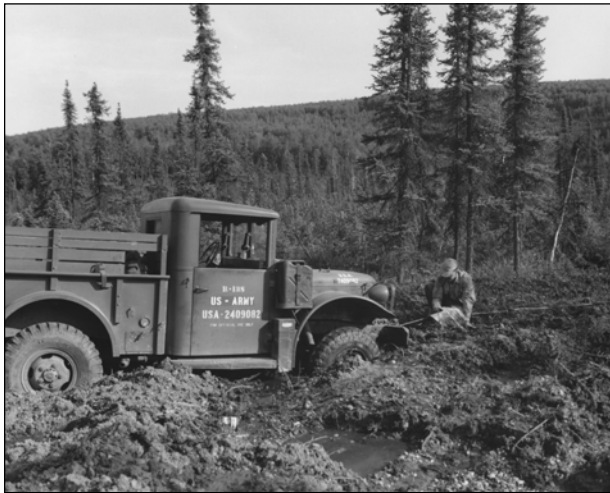
Figure 1. 10 Aug. 1954. Haines-Fairbanks POL pipeline area #3 (Harding Lake Area). Resident Engineer vehicle M-37 stuck in the mud – looking south. NARA.
