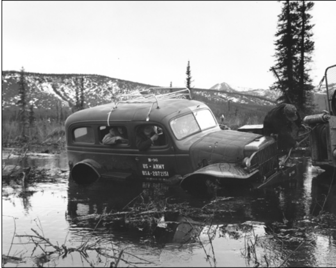
Figure 8. Area 2. Mile 1173, Yukon Territory, Corps of Engineers inspection vehicle mired along pipeline right-of-way. NARA.
