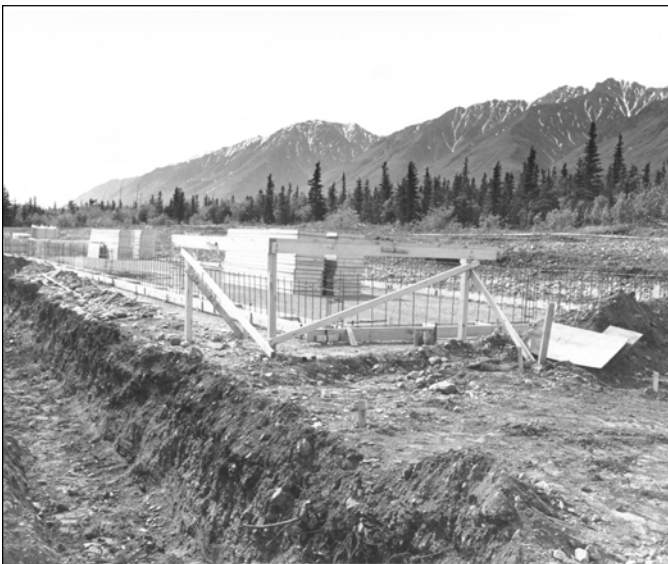
Figure 32. Destruction Bay under construction. NARA.
