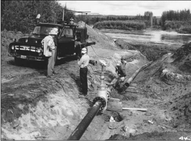
Figure 5. Laying pipe for underwater crossing. NARA, A4-3826.
