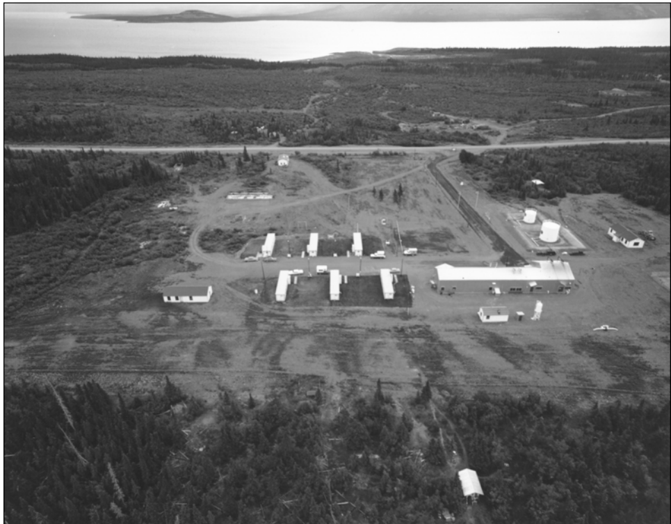
Figure 34. Destruction Bay Pump Station. NARA.
