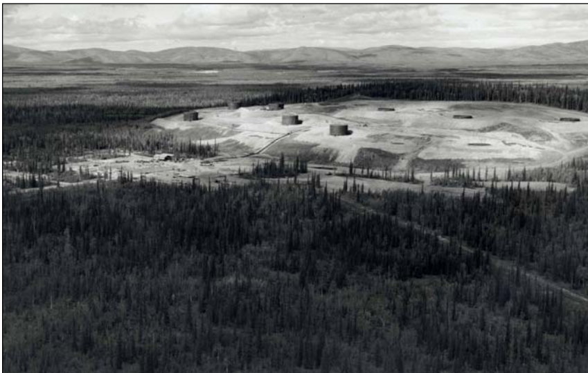
Figure 9. Tok terminal under construction, 1954. NARA.
