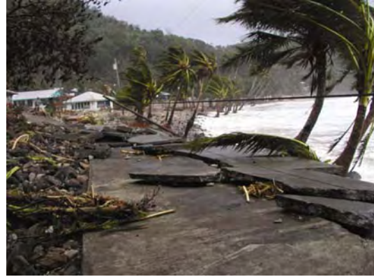
Damage to Onenoa in 2004 (Cyclone Heta).
